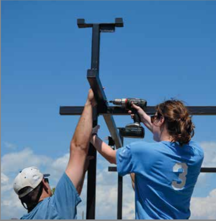
Greenville Bark Park construction
