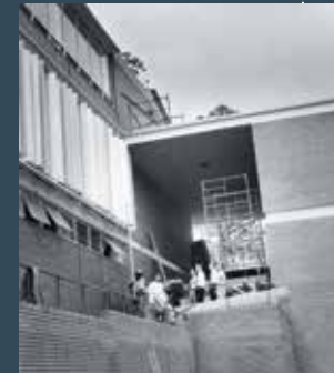
Lee Hall under construction, 1956
