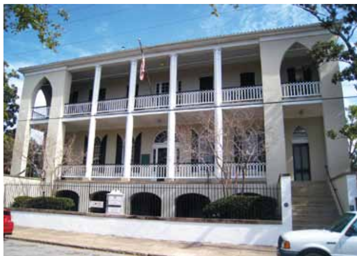
The Charleston center, currently located in Charleston's historic Marine Hospital
