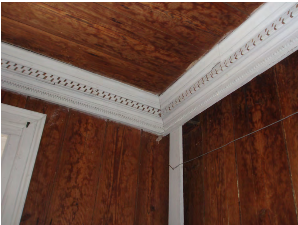
Fig. 1-20: Molding Detail from Master Bedroom
