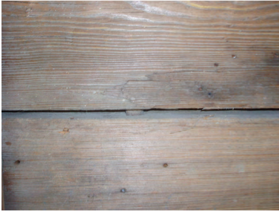
Fig. 5-9: Detail showing the peg holding two planks of the wall together.
