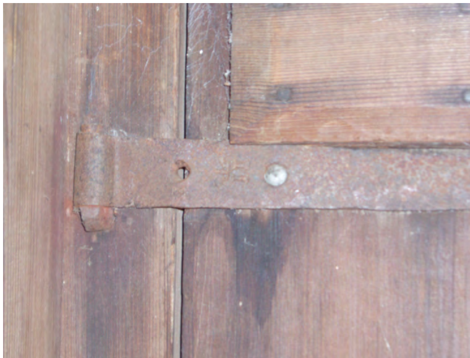
Fig. 4-14: Detail of Hinge with the Mark of the Crown from Parlor Room
