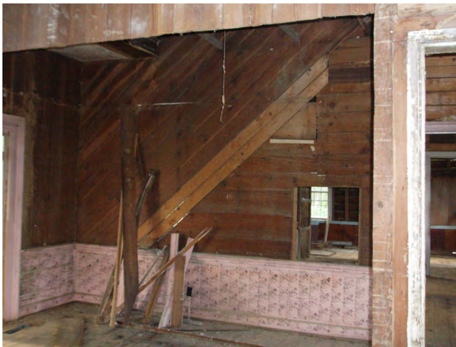
Fig. 11-9: Center Passage with ghost marks of staircase.
