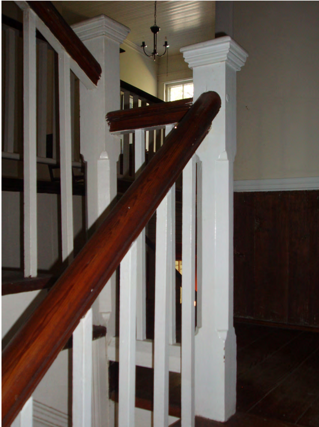
Fig. 21-12: Staircase Post with the chamfered edge and lambs tongue
