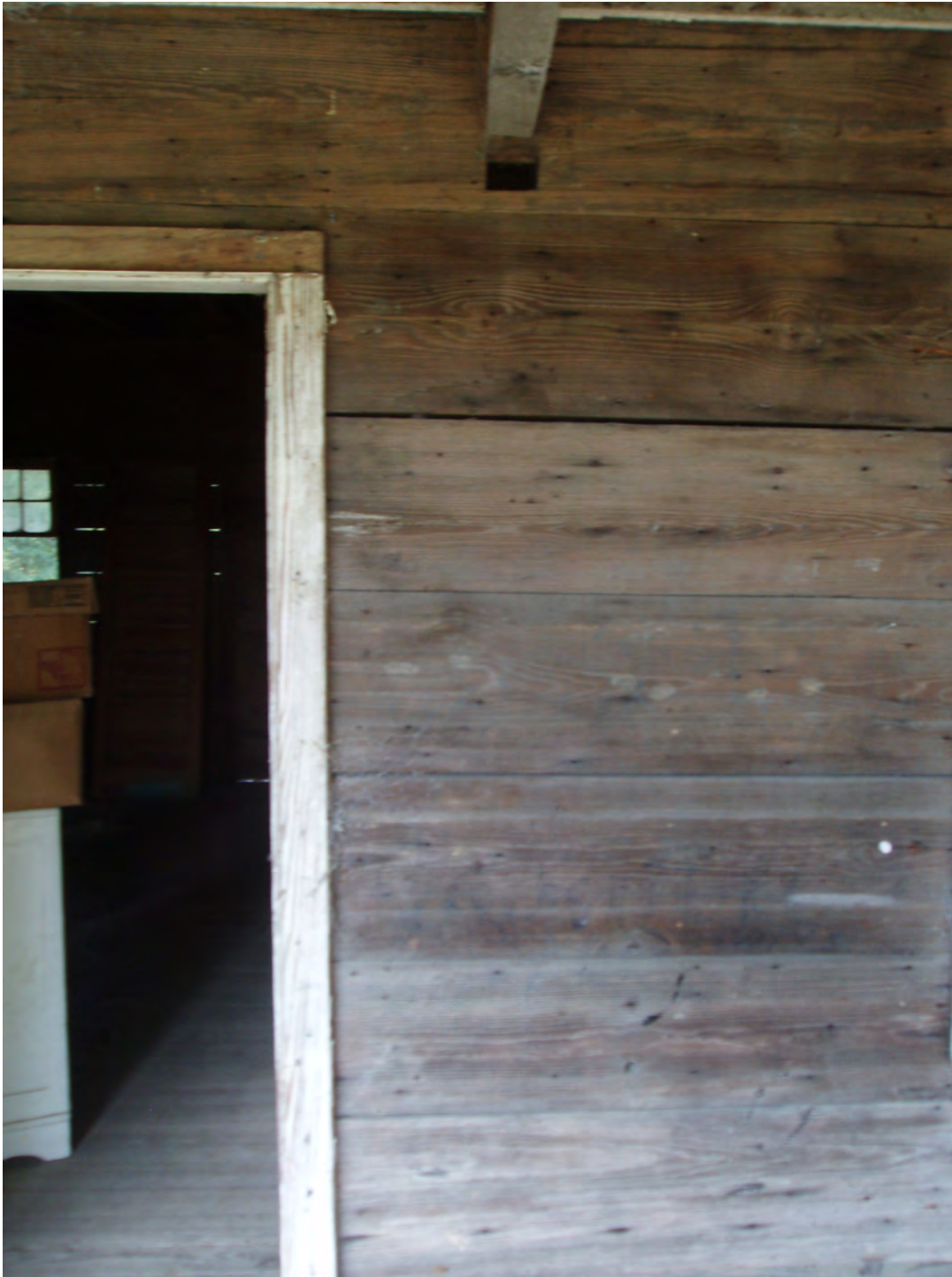
Fig. 5-8: Detail of front door jam and the wood planks for walls
