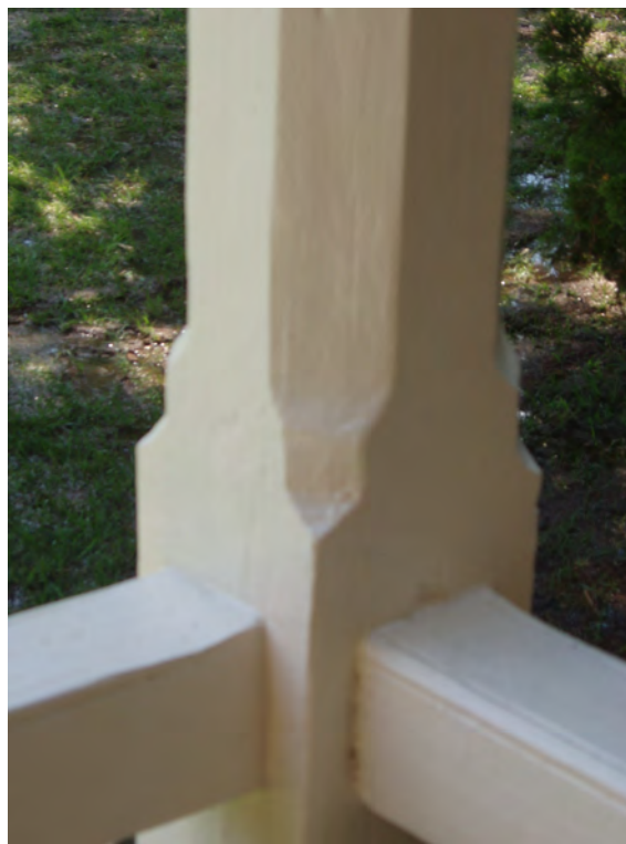
Fig 1-12: Porch Post Detail
