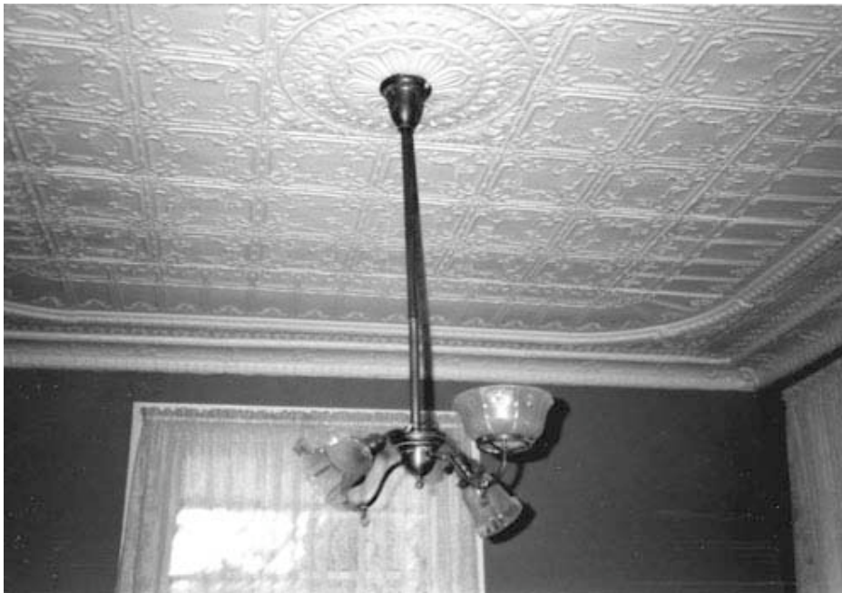
Fig. 20-6: Pressed-Metal Ceiling and Gasolier in Parlor
