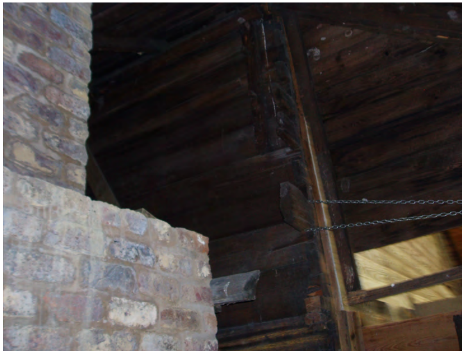
Fig. 5-7: Interior detail showing corner of log cabin construction
