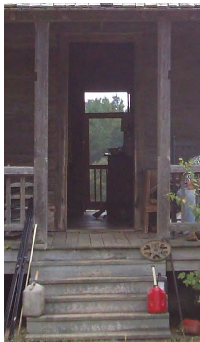
Fig. 4-18: Detail of porch posts with notches for roof extension over steps.
