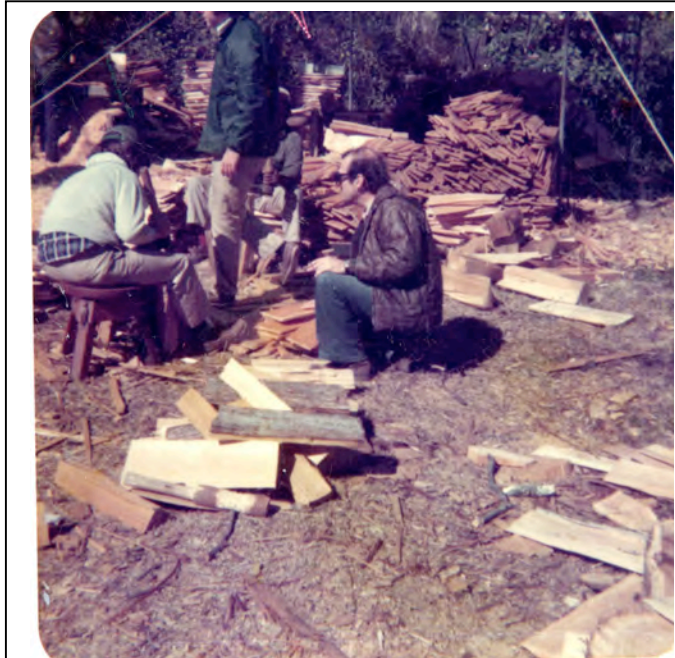
Fig. 3-17: Cypress Shingles Being Made
