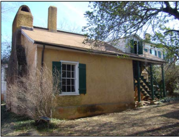
Figure 80. The west façade of the dairy/kitchen building. (Photo: Author)
