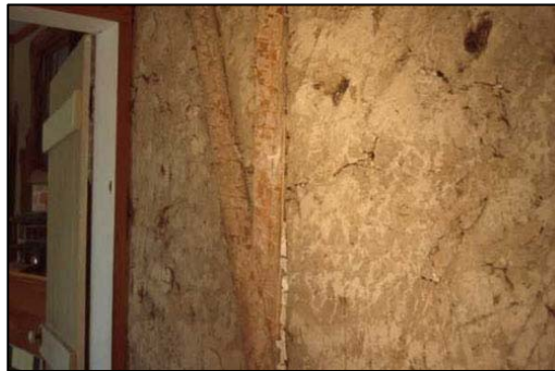
Figure 4. A bousillage wall at the Millet House in Louisiana. (Photo: www.louisianafolklife.org )
