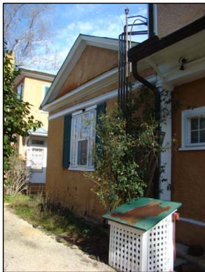
Figure 76. The northern pisé wing of the Borough House. (Photo: Author)
