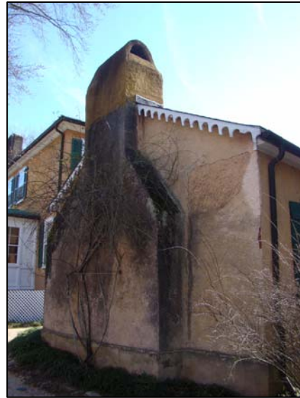
Plate 81. The north façade of the dairy/kitchen building. (Photo: Author)
