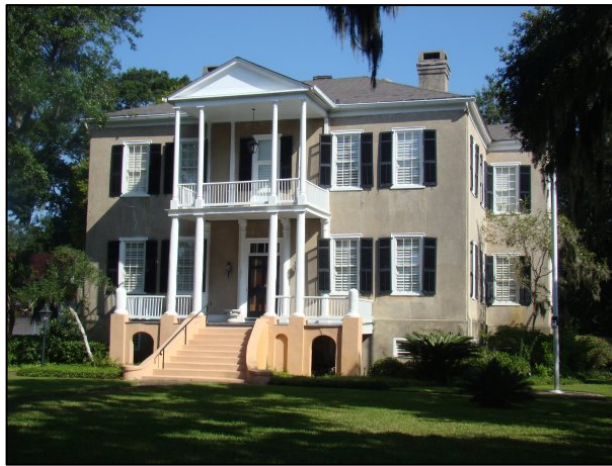
Figure 18. Tabby Manse, c. 1786, in Beaufort, South Carolina, which is built of Oglethorpe tabby. (Photo: Author)
