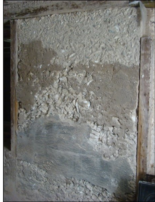
Figure 17. Tabby foundation in a house in Beaufort, South Carolina. (Photo: Author)
