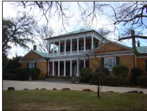
Figure 55. The Borough House with pisé wings. (Photo: Author)
