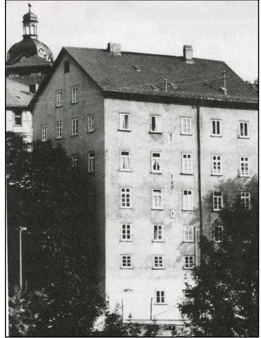
Figure 43. A seven story apartment building of pisé on a hillside built by Wimpf. (Image: Louis Cellauro and Gilbert Richaud)
