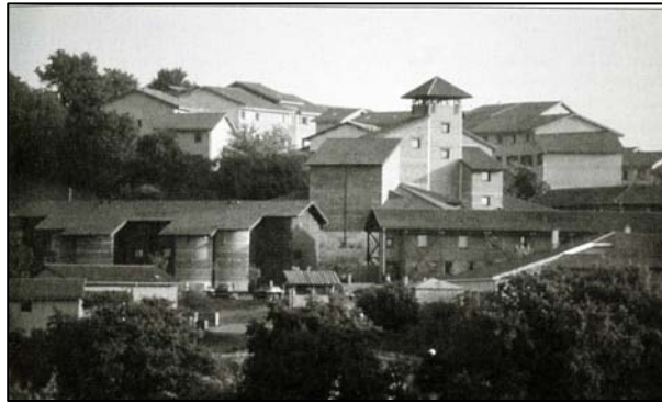
Figure 10. Modern rammed earth houses built in France. (Image: David Easton)
