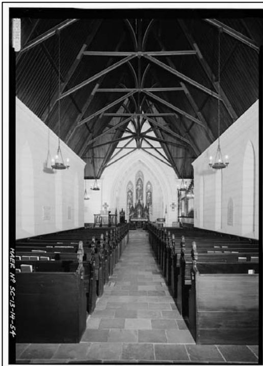
Plate A17. View looking east from the nave. (Photo: Library of Congress)
