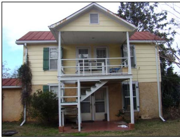
Figure 91. The cook’s house, which now serves as the caretaker’s house. It originally consisted of two stories, the bottom of pisé, and the top of wood. The wing to the left and an ell addition to the rear were built in the 1970s. (Photo: Author)
