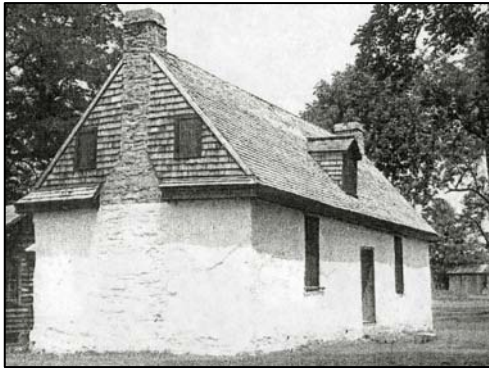
Figure 51. Pisé overseer's cabin at Pea Hill Plantation. It now serves as the entrance to Kennon House Restaurant. (Image: Gardiner Hallock)
