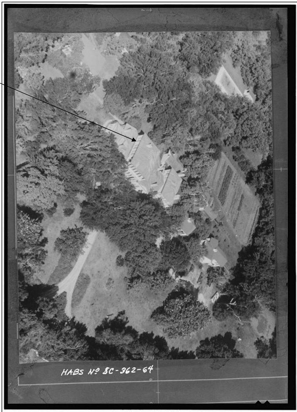
Plate A11. Aerial view of the Borough House property from 1985. (Photo: Library of Congress)
