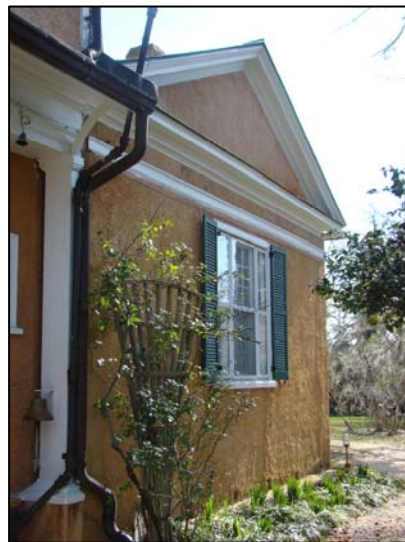
Plate 77. The southern pisé wing of the Borough House. (Photo: Author)
