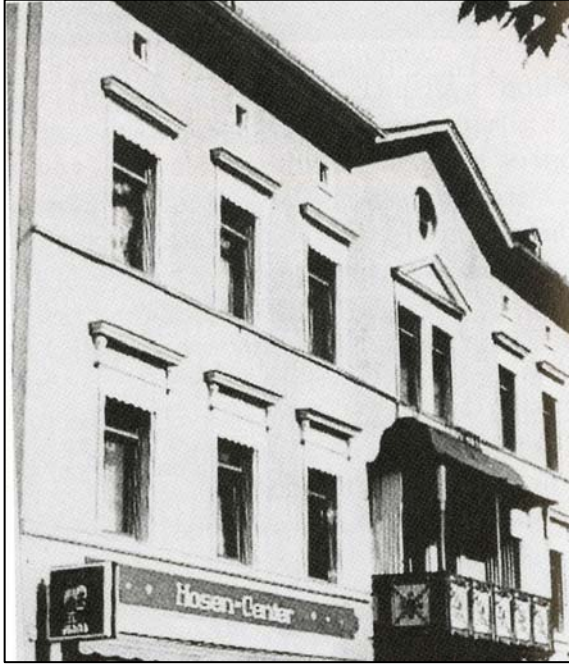
Figure 5. A townhouse designed and built by Wimpf in Weilburg an der Lahn. (Image: Louis Cellauro and Gilbert Richaud)
