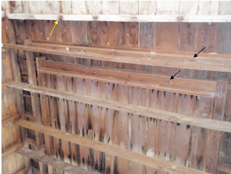
Figure 5.50: Evidence of past walls can be seen on the ceiling. The black arrows are pointing to rows of mortises that follow the square in the ceiling. These are from a double wall construction that surrounded the ice pit. The yellow arrow points to the row that would have separated the one room into two. The whitewash in the front portion also shows what was once two spaces. (Photo by Author, 2009)
