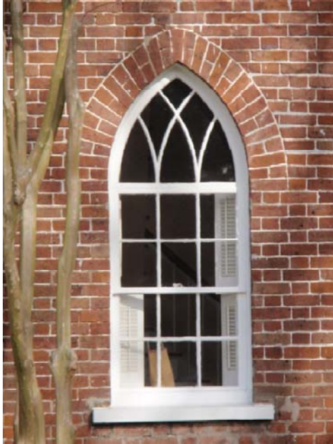
Figure 5.63: Example of the first floor, double-hung, lancet windows. (Photo by Author, 2010)
