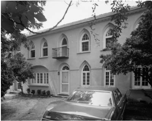
Figure 5.5: Photo of the carriage house at 110 Broad Street.
