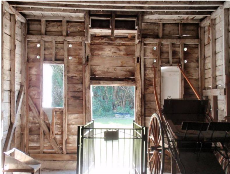
Figure 5.52: Interior view of the south elevation. (Photo by Author, 2009)
