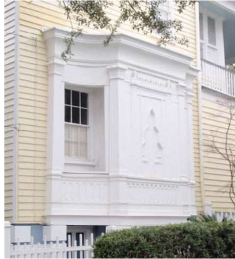
Figure 4.13: Gothic detailing on the Bennett/Jones House at 89 Smith Street. Ca. 1840. (Photo by Author, 2010)
