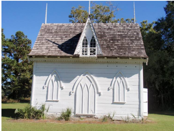
Figure 5.44: West elevation of the ice house with the blind lancet windows on the side. (Photo by Author, 2009)
