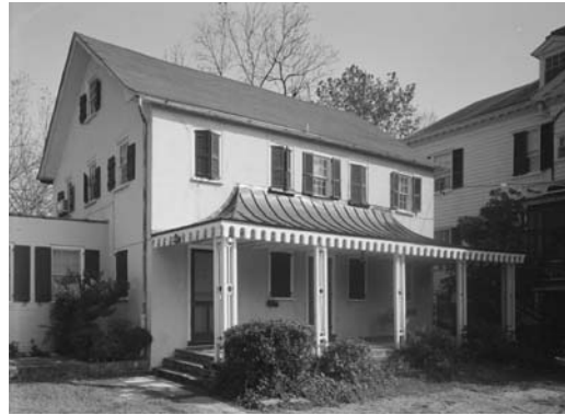
Figure 5.35: The kitchen at 60 Montagu Street ca. 1977. (Library of Congress, Prints and Photographs Division, Historic American Buildings Survey, HABS SC,10-CHAR,283A-, http://hdl.loc.gov/loc.pnp/hhh.sc0586 )
