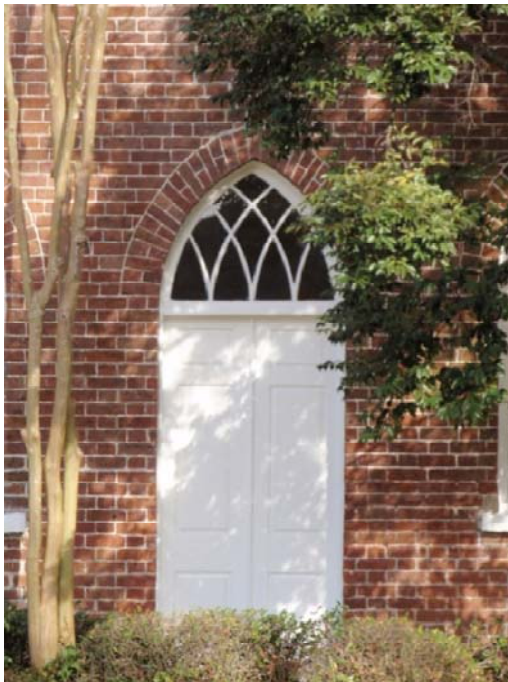
Figure 5.65: Exterior view of door in the west elevation. (Photo by Author, 2010)
