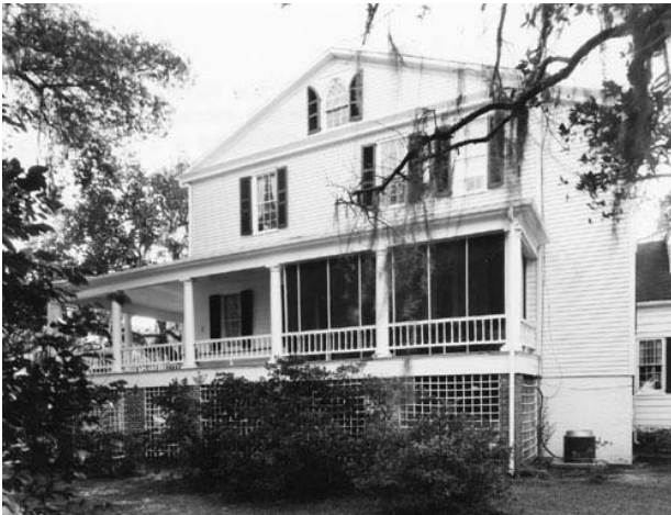
Figure 4.25: Chicora Wood Plantation, Right Elevation, Note the small lancet window under the peak of the roof. Built before 1819.
