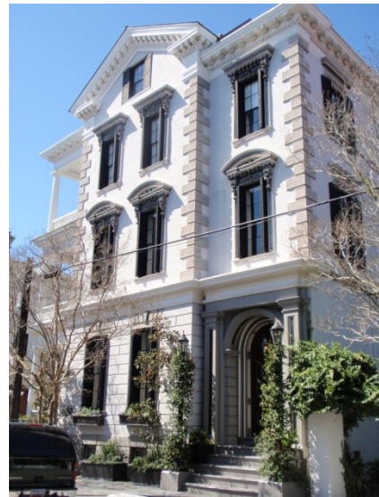
Figure 5.17: The main house at 21 King Street done in the Italianate style. (Photo by Author, 2010)
