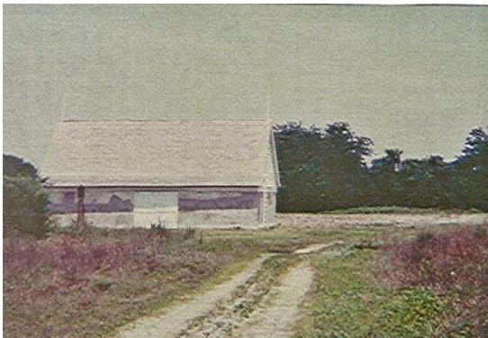
Figure 5.42: 1967 Photo of the tabby stable taken by Mrs. Legare Head. It has Gothic Revival trim.
