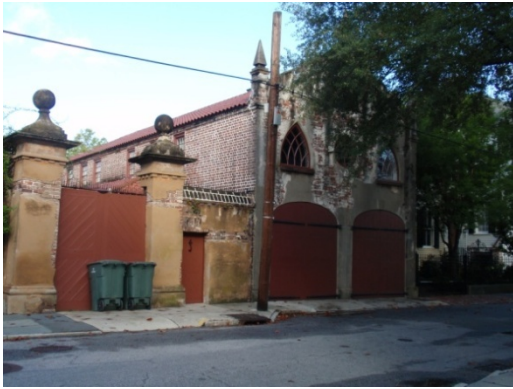
Figure 6.7: Photo of 27 King with the front façade of the carriage house fronting the street. (Photo by Author, 2009)
