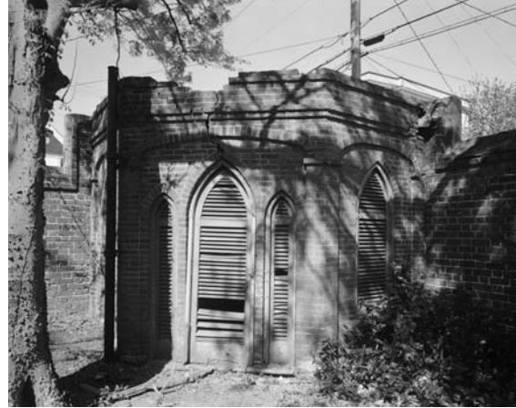
Figure 5.79: One of two privies located in the northwest and northeast corners of the yard, 1979. (Library of Congress, Prints and Photographs Division, Historic American Buildings Survey, HABS SC,10-CHAR,177D-3, http://hdl.loc.gov/loc.pnp/hhh.sc0024 )
