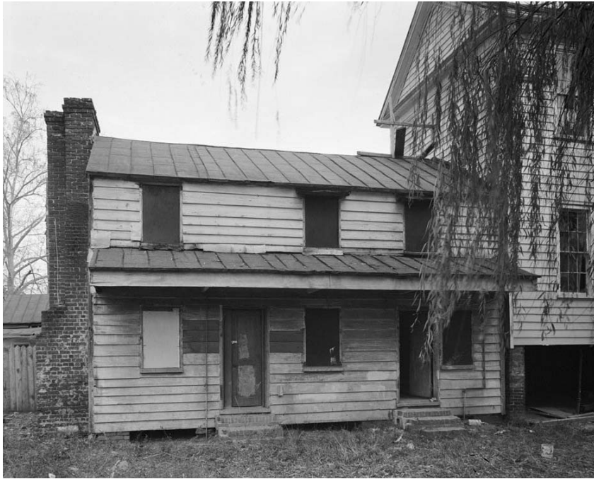
Figure 3.7: 8 Judith Street, a typical wooden outbuilding.
