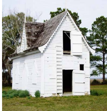
Figure 5.41: Photo of the icehouse showing the ladder in place which is no longer there.
