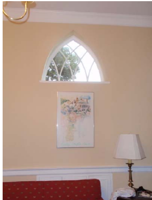
Figure 5.66: Interior view of the door in figure 5.55. The door has been blocked from the inside with only the window in view. (Photo by Author)
