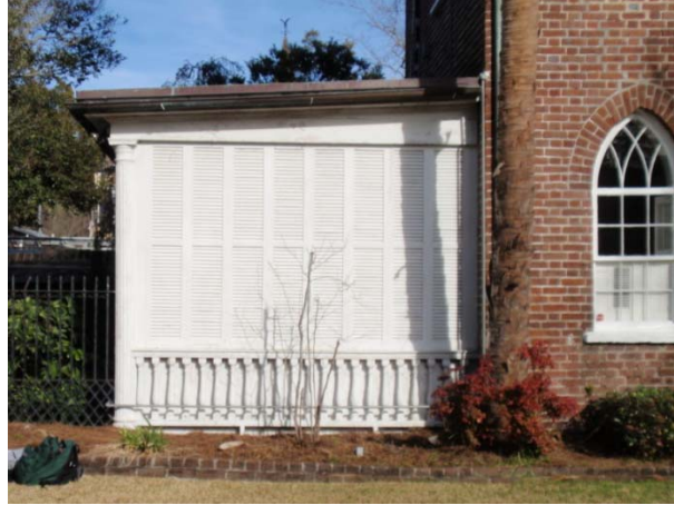
Figure 5.68: The wooden addition on the north end of the building. The railing and corner post of the original porch that has been closed in can be seen. (Photo by Author, 2010)
