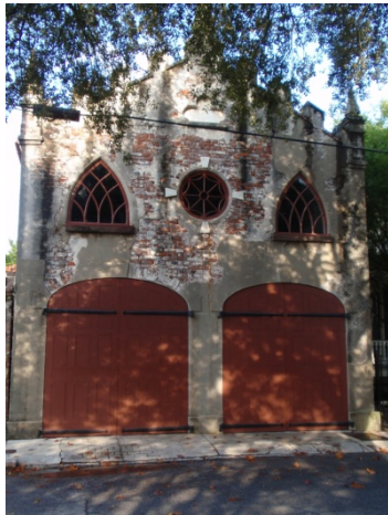
Figure 5.18: The front of the carriage house today at 27 King Street. (Photo by Author, 2009)
