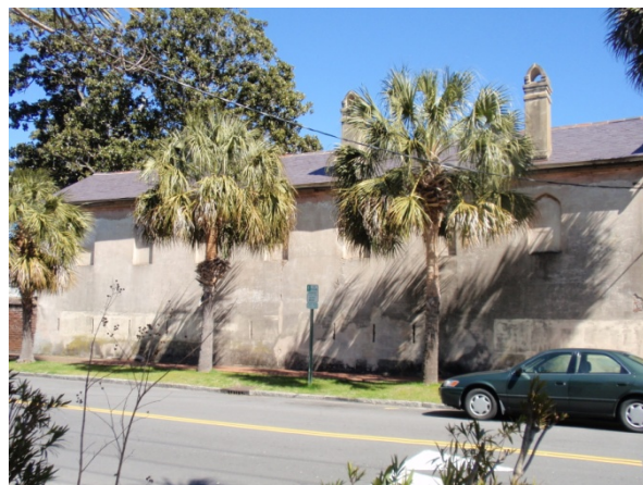
Figure 6.12: View of the arches on the outside of the Aiken-Rhett (48 Elizabeth Street) stable from the street. (Photo by Author, 2010)
