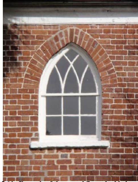
Figure 5.64: Example of the second floor, double-hung, lancet windows. (Photo by Author, 2010)
