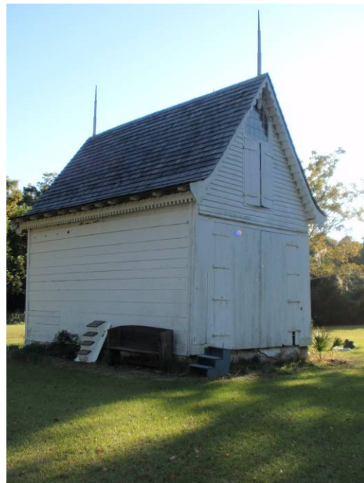
Figure 5.46: The north and east sides of the building. The north side of the building has a large door that opens with a smaller one in the gable. A divided light window can be seen above. The east side of the building has no added details other than the trim along the eave. (Photo by Author)
