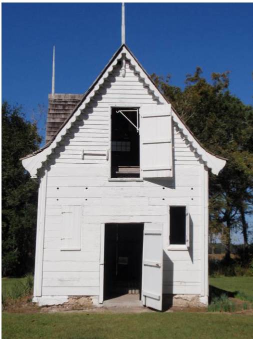
Figure 5.45: South elevation of the ice house with its door and two windows. The bellcast roof and bargeboard trim can be seen. To the left of the door opening into the gable can be seen the wooden bar for attaching a ladder. The tabby foundation has been exposed where it has begun chipping away. (Photo by Author, 2009)
