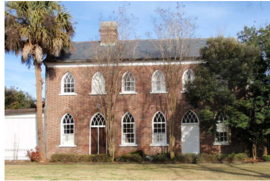
Figure 5.56: West elevation of the carriage house at 18 Bull Street today. (Photo by Author, 2010)
