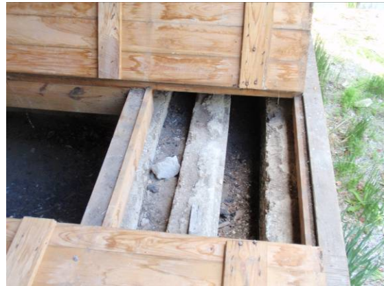
Figure 5.54: Photo showing the differing layers of tabby construction making up the foundation and the ice pit. (Photo by Author, 2009)
