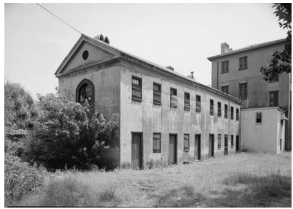
Figure 5.73: The west elevation of the kitchen building, 1962. (Library of Congress, Prints and Photographs Division, Historic American Buildings Survey, HABS SC,10-CHAR,177C-2, http://hdl.loc.gov/loc.pnp/hhh.sc0026 )
