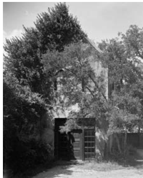
Figure 5.13: South Elevation. 1977 photo. (Library of Congress, Prints and Photographs Division, Historic American Buildings Survey, HABS SC,10-CHAR,123A-2, http://hdl.loc.gov/loc.pnp/hhh.sc0711 )
