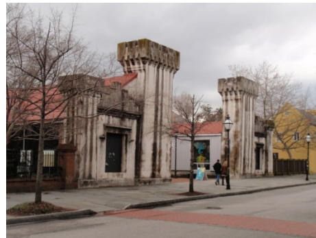
Figure 4.9: South Carolina Railroad Complex gates. (Photo by Author, 2010)
