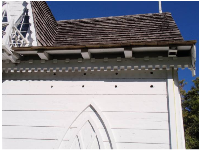
Figure 5.47: Detail of the trim on the eaves. Holes to provide ventilation to the front portion of the ice house can clearly be seen. (Photo by Author, 2009)
