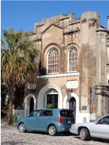
Figure 4.12: The German Fire Steam Engine Company at 8 Chalmers Street. Built 1851. (Photo by Author, 2010)
