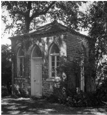
Figure 5.57: The gazebo behind 18 Bull Street. Photo taken 1977-78. (Library of Congress, Prints and Photographs Division, Historic American Buildings Survey, HABS SC,10-CHAR,130C-2, http://hdl.loc.gov/loc.pnp/hhh.sc0059 )
