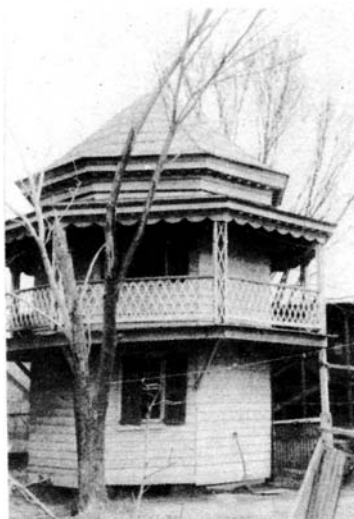
Figure 6.15: Small Building that was at 91 Beaufain Street. (In Samuel Gaillard Stoney, This is Charleston: A Survey of the Architectural Heritage of A Unique American City Undertaken by the Charleston Civic Services Committee , (Charleston, SC: The Carolina Art Association, 1944), 9.)
