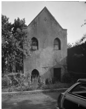
Figure 5.12: North Elevation. 1977 Photo. (Library of Congress, Prints and Photographs Division, Historic American Buildings Survey, HABS SC,10-CHAR,123A-2, http://hdl.loc.gov/loc.pnp/hhh.sc0711 )
