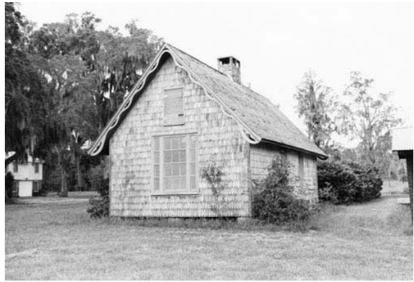
Figure 4.26: Annandale Plantation, Outbuilding-Slave Cabin, Georgetown County. (South Carolina Department of History and Archives, National Register Property Listings, http://www.nationalregister.sc.gov/georgetown/S10817722007/index.htm )
