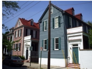
Figure 3.2: Typical Charleston single houses.
