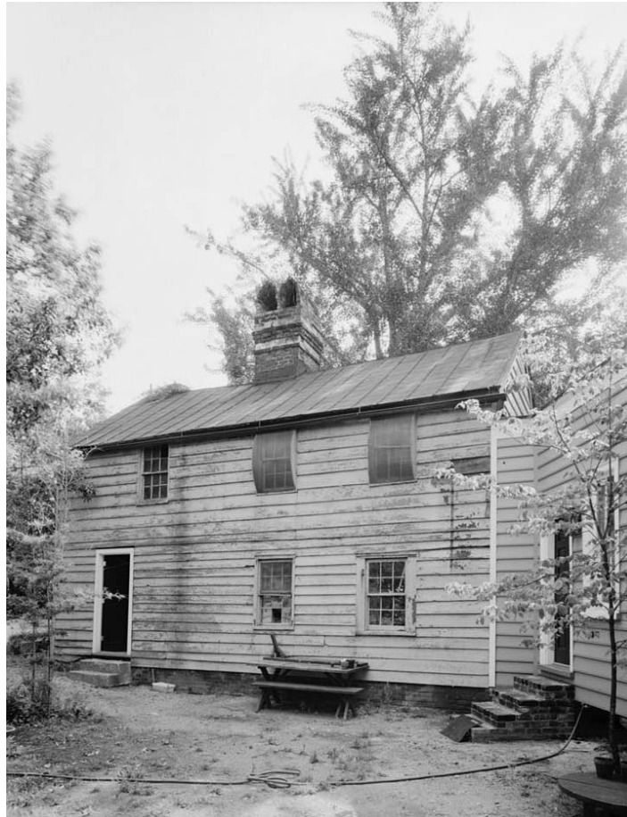
Figure 3.4: 126 Tradd Street outbuilding. Early 18th century layout with the chimney in the middle. Library of Congress, Prints and Photographs Division, Historic American Buildings Survey, HABS SC,10-CHAR,322A-1, http://hdl.loc.gov/loc.pnp/hhh.sc0545 (accessed February 10, 2010).
