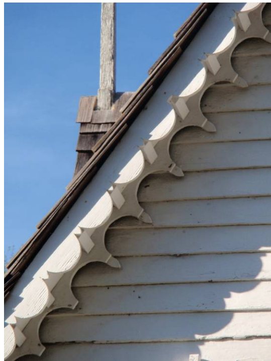
Figure 5.49: The trim on the end of the gable roofs. (Photo by Author, 2009)
