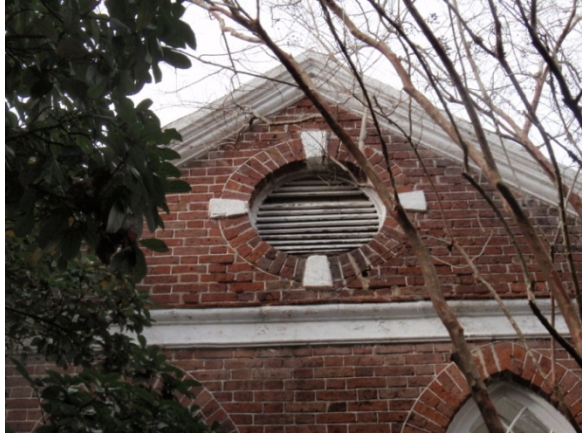
Figure 5.67: Details in the roof gable. (Photo by Author, 2010)
