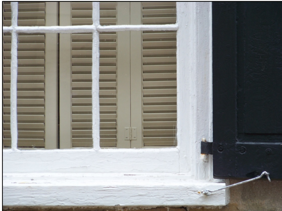
FIG. 6-5: CLOSE-UP OF EXISTING HISTORIC WINDOW AT 15 HARBOR STREET. PHOTOGRAPH BY AUTHOR. 3 MAR. 2010.
