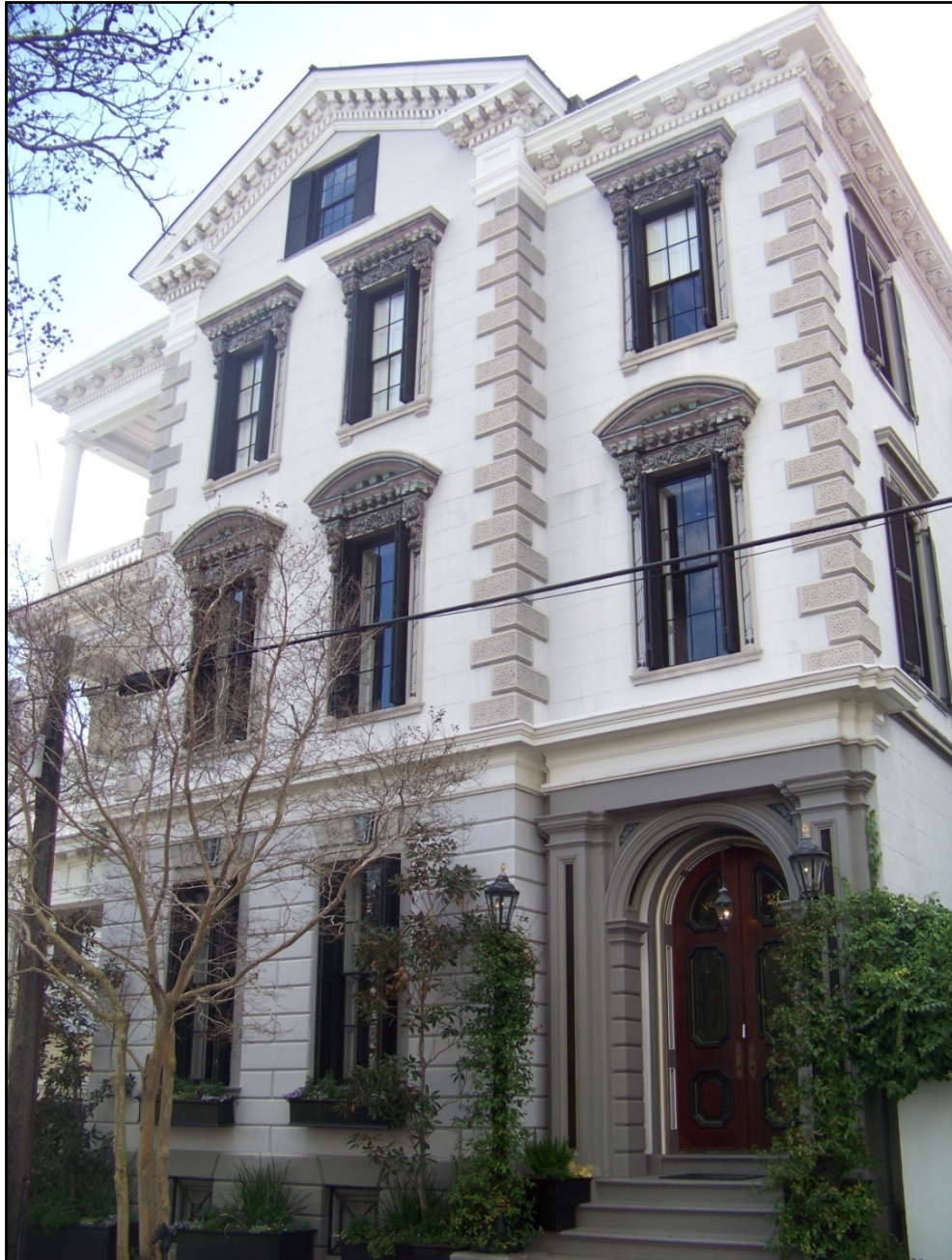
FIGURE I.20 21 KING STREET, CHARLESTON, SC. PHOTOGRAPH BY AUTHOR. 15 MAR. 2010.
