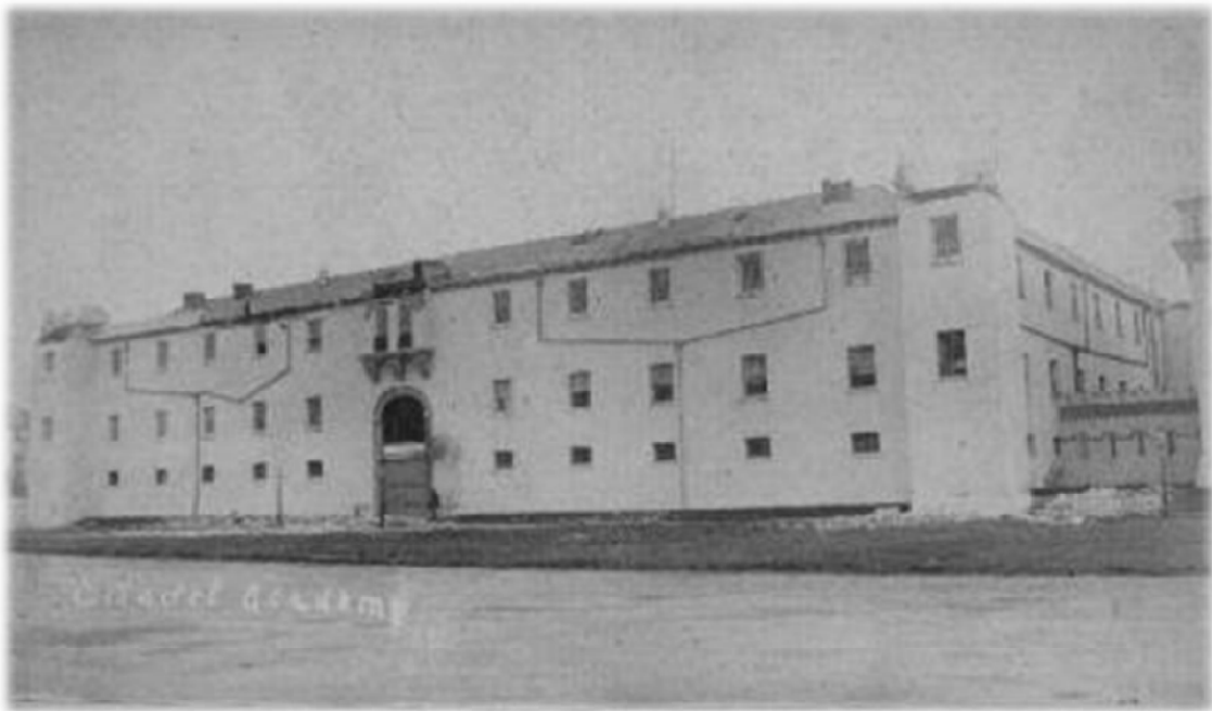
Fig. 4.12 Photograph of the Old Citadel after the 1886 earthquake
