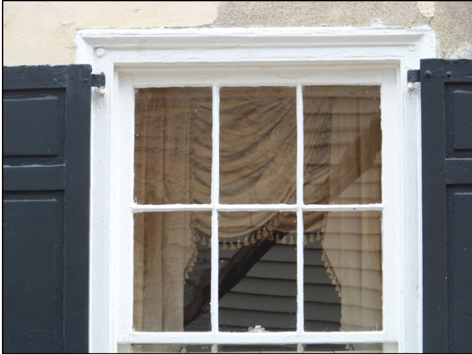
FIG. 6.4 CLOSE-UP OF EXISTING HISTORIC WINDOW AT 15 HARBOR STREET. PHOTOGRAPH BY AUTHOR. 3 MAR. 2010.
