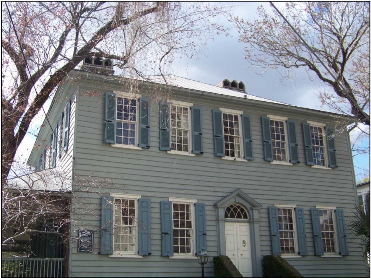
FIGURE I.14 19 ARCHDALE STREET, CHARLESTON, SC. PHOTOGRAPH BY AUTHOR. 15 MAR. 2010.
