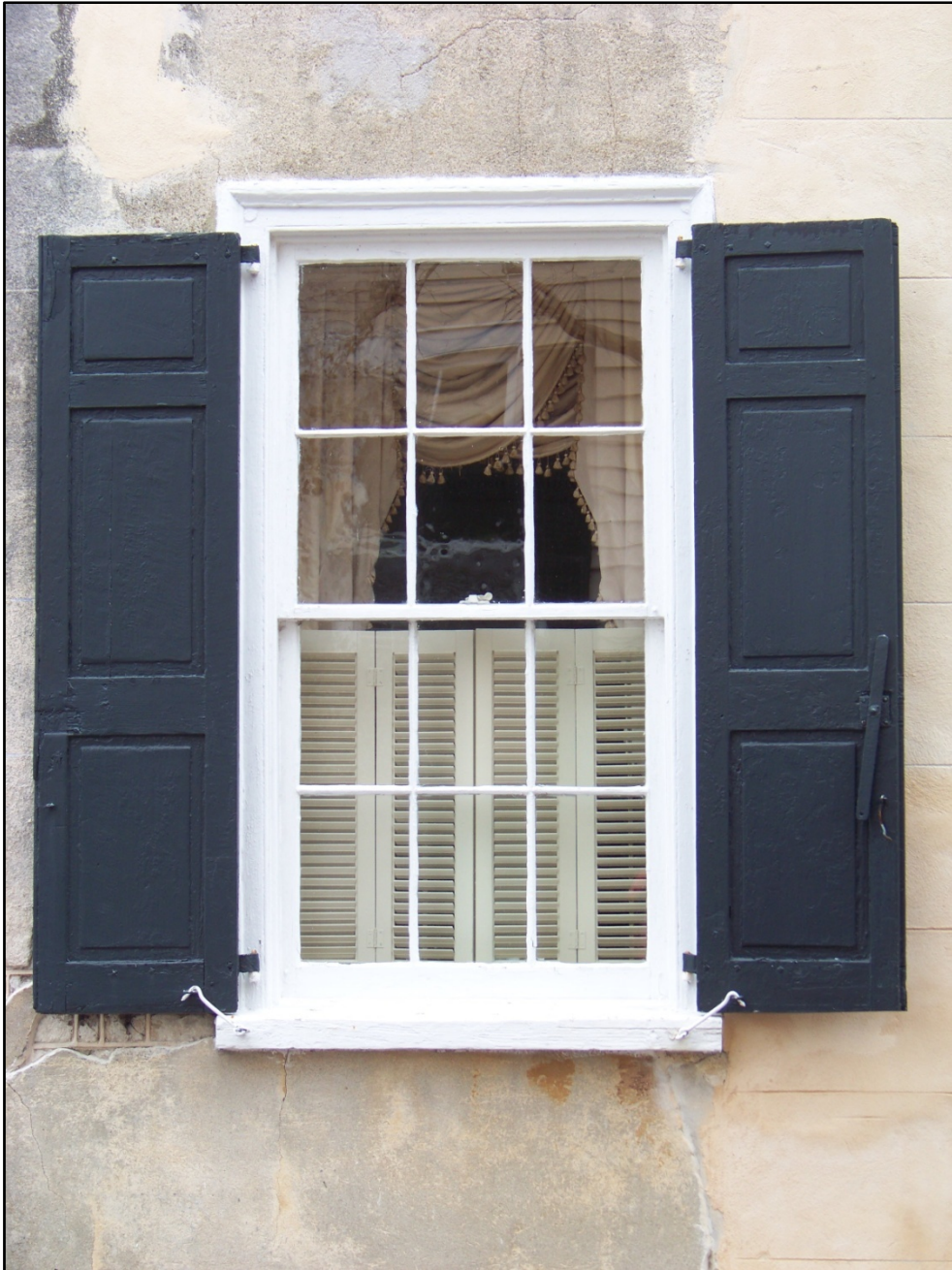
FIG. 6.3 CLOSE-UP OF EXISTING HISTORIC WINDOWS AT 15 HARBOR STREET. PHOTOGRAPH BY AUTHOR. 3 MAR. 2010.
