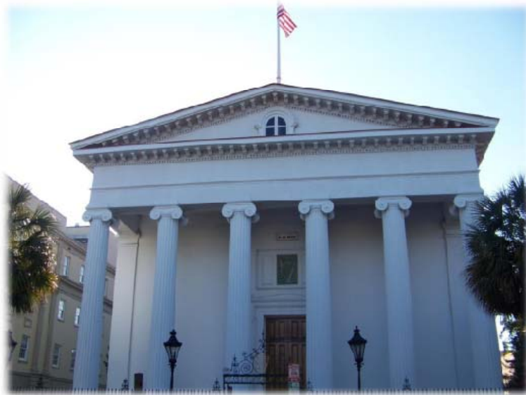
Fig. 1.8 Hibernian Hall (Constructed 1840) 105 Meeting Street
