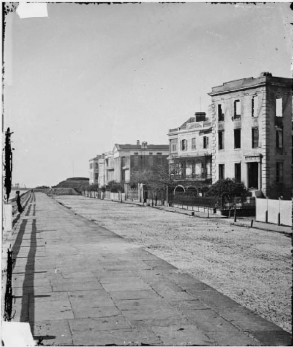
(Left) Fig. 4.7 A house that has been burnt out at the corner of Atlantic and East Bay Photograph taken in April 1865
