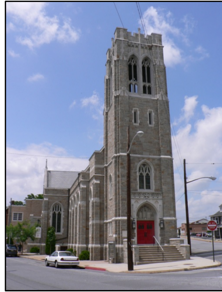
Fig. 2, above. A modern photograph of the front (east) elevation (Photo by author). Fig. 3, below. Exterior materials of the building are Plymouth stone and cast concrete (Photos by author).
