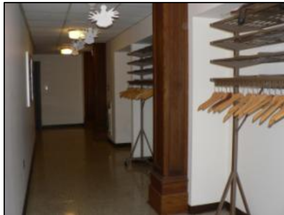
Fig. 4, above. Interior spaces which were once divided by moveable walls have been replaced with permanent walls; however the outline of original openings can still be determined (Photo by author). Fig. 5, below. The original decorative wood columns which skirted the second-floor balcony are retained between the subdivided spaces (Photo by author).
