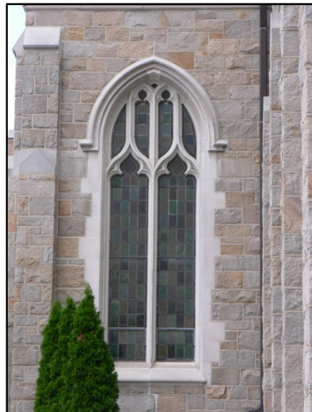
Fig. 2, above. A modern photograph of the front (east) elevation (Photo by author). Fig. 3, below. Exterior materials of the building are Plymouth stone and cast concrete (Photos by author).
