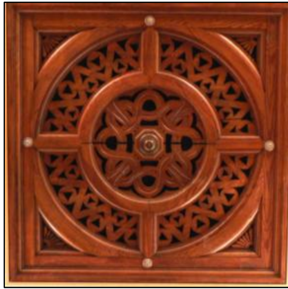
Fig. 5. One of the many wood vents which were found and reused during the most recent renovation (Photo by author).
