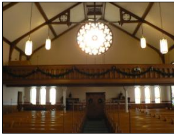
Fig. 2, above. The interior of the sanctuary looking toward the altar at the north (Photo by author). Fig. 3, below. The interior of the sanctuary looking toward the balcony at the south end; note the exposed wood trusses and vents (Photo by author).
