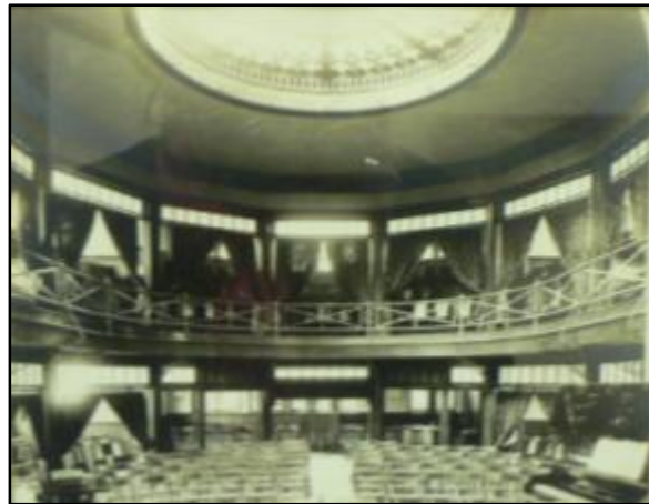
Fig. 2, above. The Sunday School wing was designed in the Akron Plan; date unknown (Photo courtesy of Dave Boyles). Fig. 3, below. A majority of the Dempwolf-designed details have been removed or covered by drop ceilings; note the large skylight is still in place and the blue altar niche (Photo by author).
