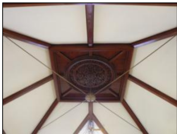
Fig. 3, above. The auditorium includes angled pews which slope down to the altar (Photo by author). Fig. 4, below: The ceiling rises to roof height and incorporates wood ribs and a large wood ceiling vent (Photo by author).
