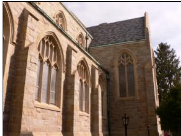
Fig. 2. The intersection of the nave and the west transept; note the tracery in the windows and the clerestory level above (Photo by author).
