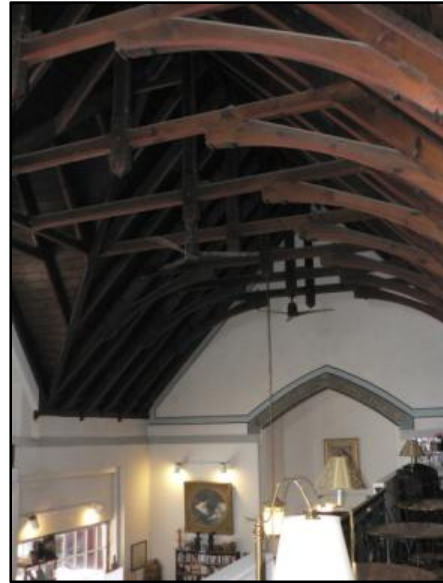
Fig. 4. The interior of the church today with original exposed trusses (Photo by author).
