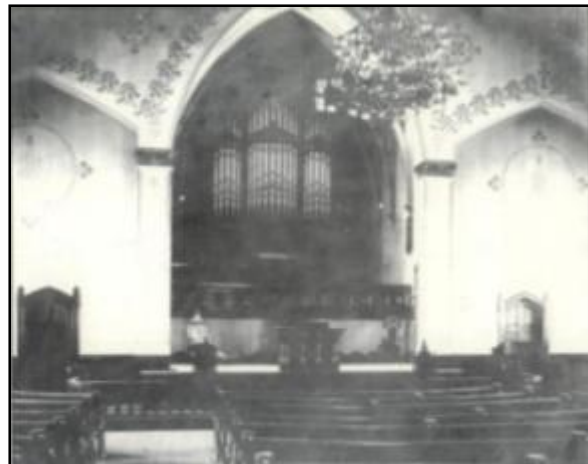
Fig. 6. St. John's Evangelical Lutheran Church located in Steelton, PA includes most of the features seen in auditorium-plan buildings: square plan, thin columns, bowled floor sloping to the altar, and a preaching stage (Photo by author). Fig. 7. St. Matthew's Lutheran Church, originally located in Hanover, PA was designed in 1878 and included a preaching platform, choir loft, and organ (St. Matthew Lutheran Church. Outline of St. Matthew's History . http://www.stmattlutheran.org/Pages/History/history_main.htm (accessed September 14, 2009).
