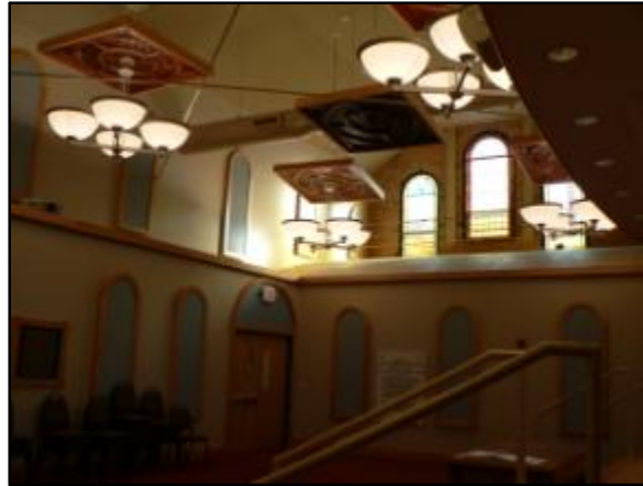
Fig. 4. The interior of the church today. The original ceiling heights were retained and windows and wood vents exposed (Photo by author).
