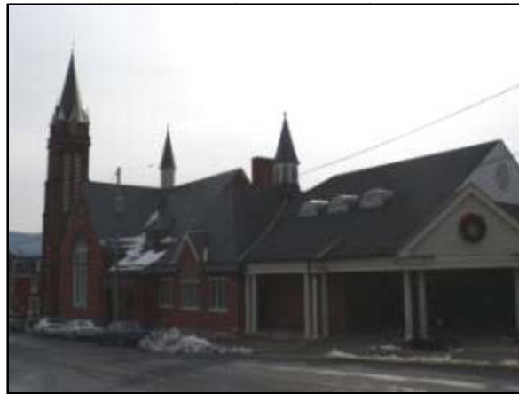
Fig. 2, above. The west side elevation shows the series of additions and renovations that occurred to the building. From south to north: the Dempwolf-designed sanctuary, the original chapel, the Dempwolf-designed Sunday school extension, a modern addition (Photo by author). Fig. 3, below. The interior of the sanctuary looking north to the altar wall (Photo by author).
