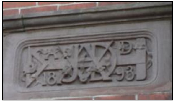
Fig. 6, above. The signature stone is dated 1893 and composed of Hummelstown brownstone (Photo by author). Fig. 7, below. The north and east (side) elevations have been significantly changed from semi-circular walls (Photo by author).
