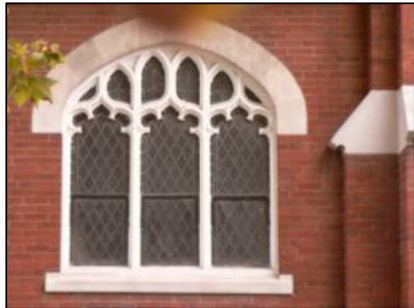
Fig. 2. The building is composed of brick with cast concrete accent elements; note the typical window which is repeated on all three elevations (Photo by author).
