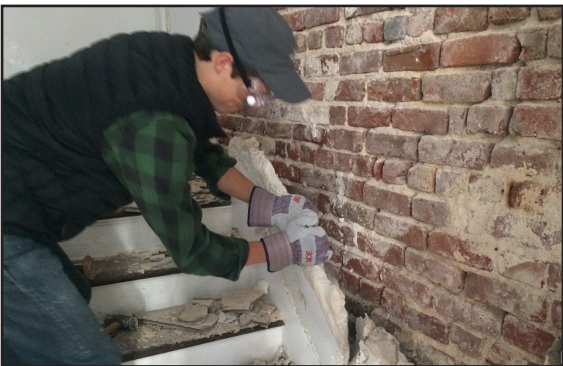
Steven Lyles removes plaster from a wall to be repointed. Image: Matt Amis.
