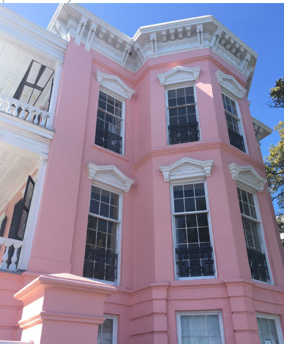
East facade of 5 East Bay Street.
