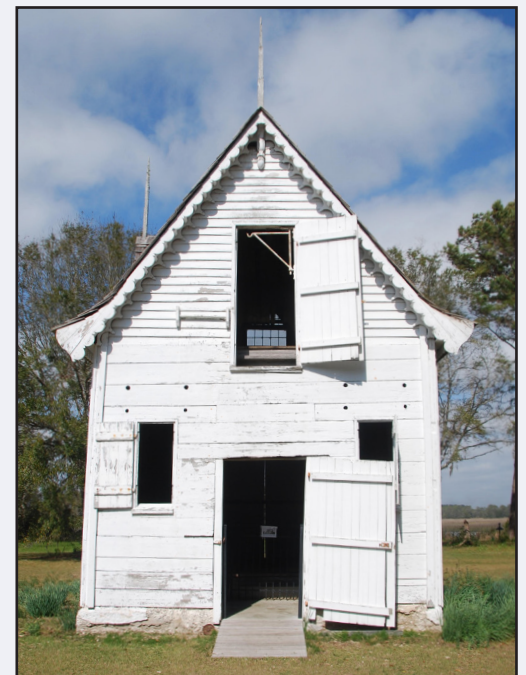
South Elevation of Icehouse. Image: Matt Amis
