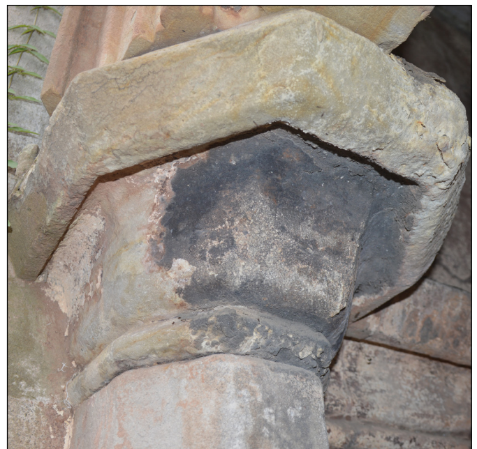
Figure 13. Black Crust on the interior of the monument.
