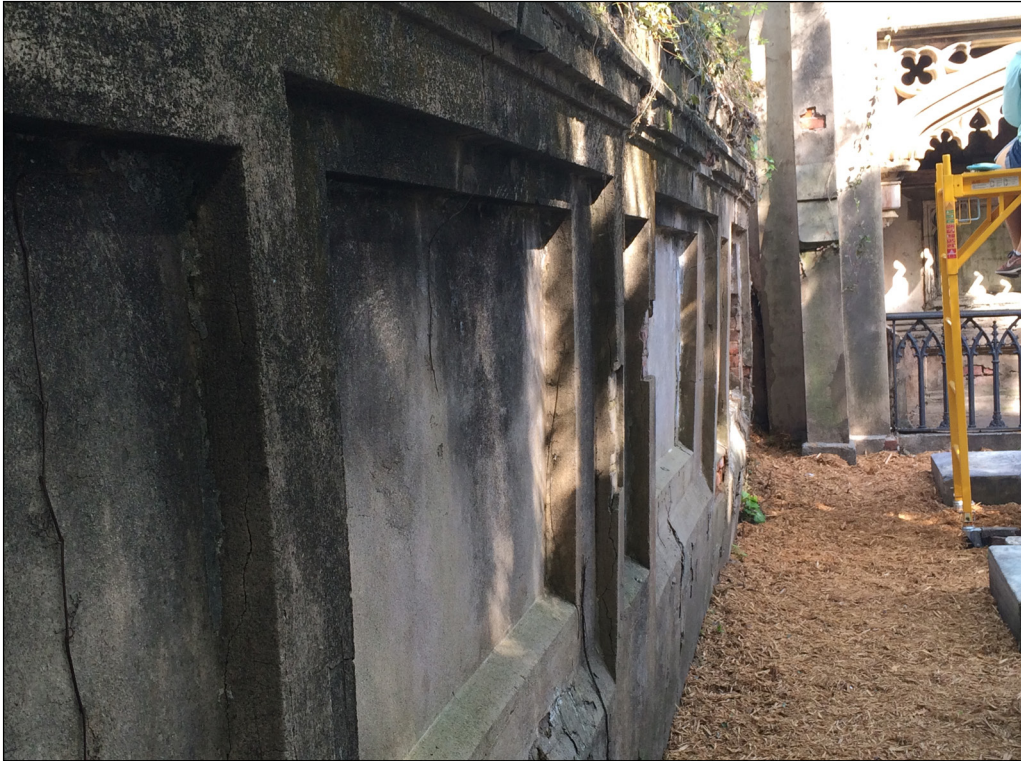
Figure 27 and 28. Bowing on the north (top) and south (bottom) sections of the west wall
