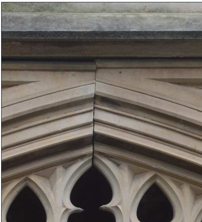
Figure 11. The shift in the center stones.
