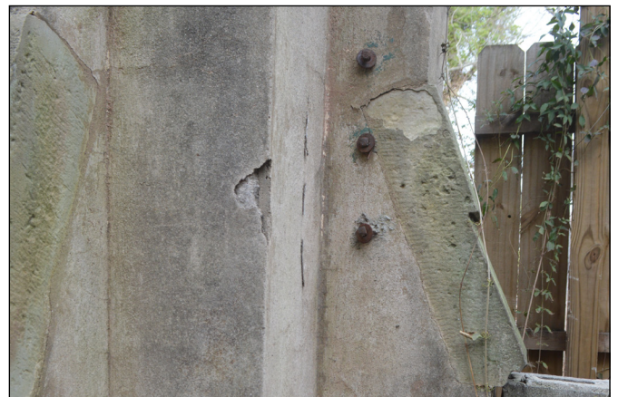
Figure 10. Bolts on the east side of the tower of unknown purpose
