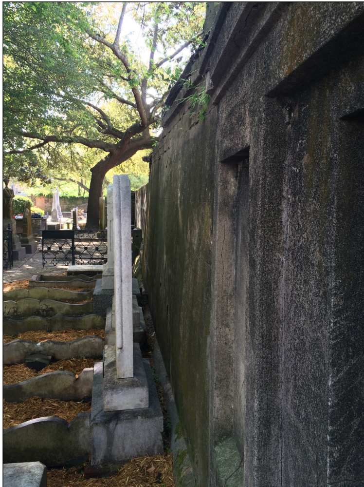
Figure 27 and 28. Bowing on the north (top) and south (bottom) sections of the west wall
