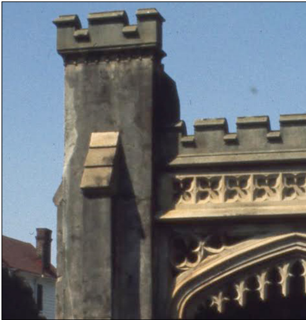
Figure 6. Historic photograph of the west tower.
