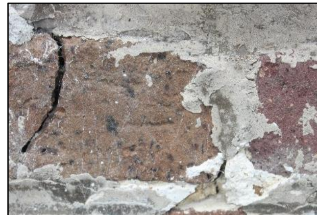
The use of Portland cement has caused bricks to crack.
