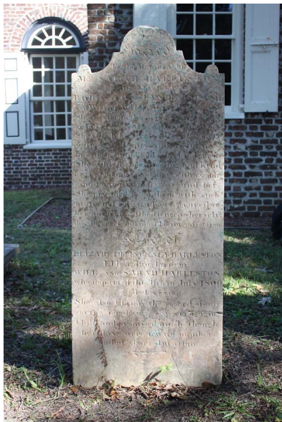
West Elevation, before cleaning. Note staining and biogrowth
