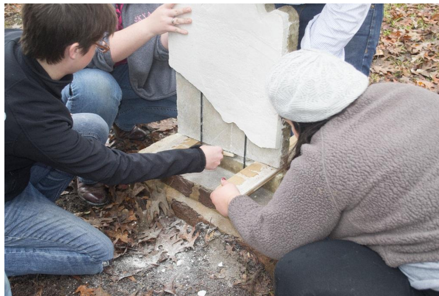
Pieces secured together with epoxy with a NHL lime and sad back. Carbon fiber rods inserted in bottom.
