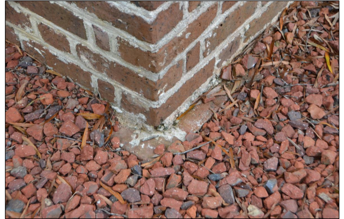
The French Drain surrounds the perimeter of the building.
