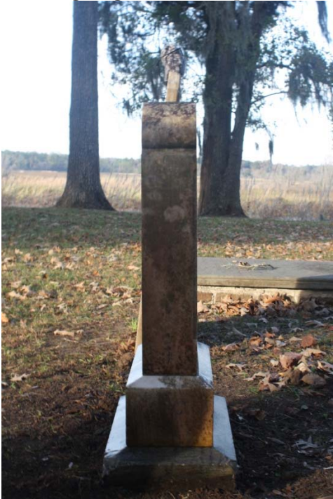
-After righting and biocide application.
