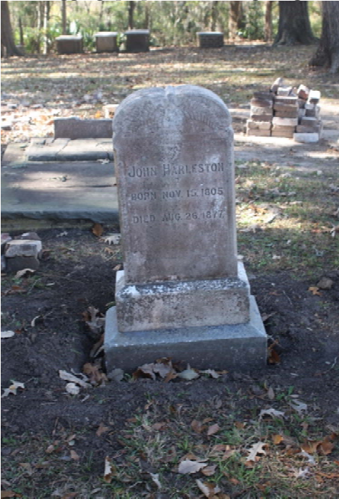
After digging/preparation for righting-
