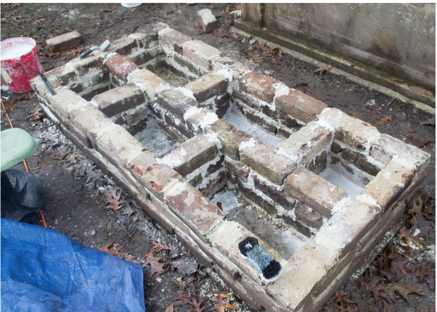
Brick built back up to form the base of the box tomb
