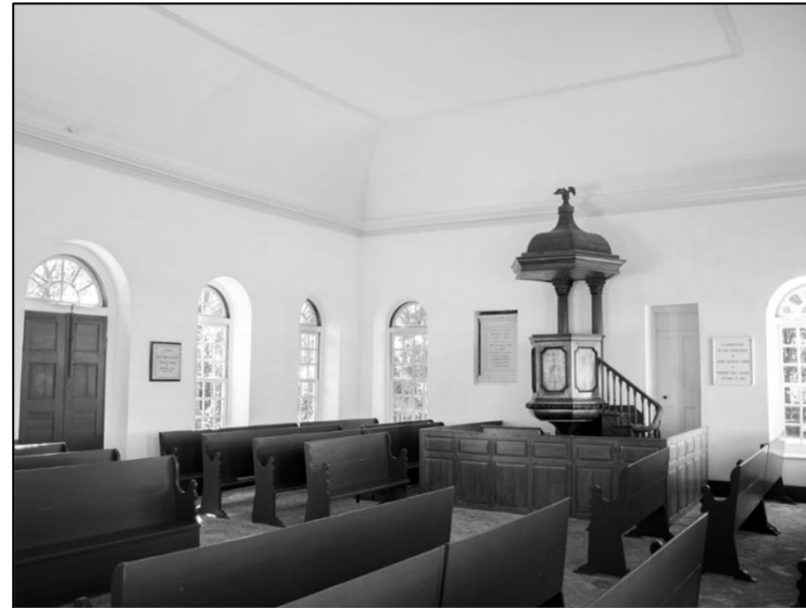
View of cornice, cove ceiling, and additional molding
