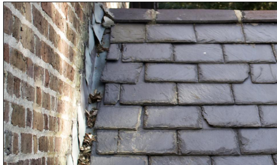
A detail of the flashing on the vestry.
