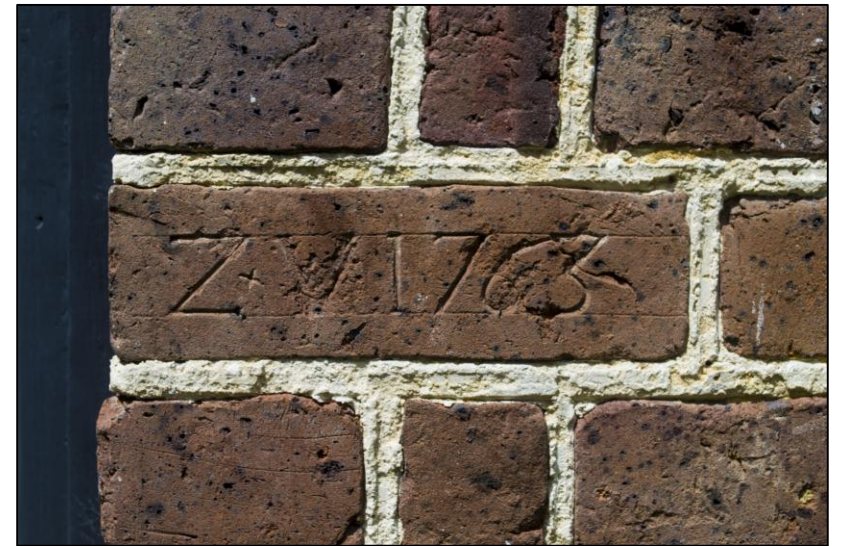
Mason Mark bricks are visible on the building near the doorways. There is also some 'historic graffiti' on the structure, occurring mostly behind shutters.
