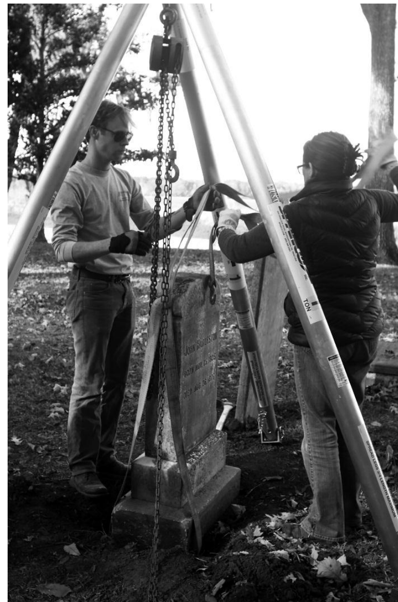
Lifting the Stone with Crane
