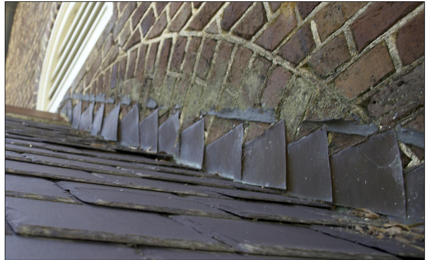
A detail of the flashing on the chancel. This shows the arch supporting the bay below.
