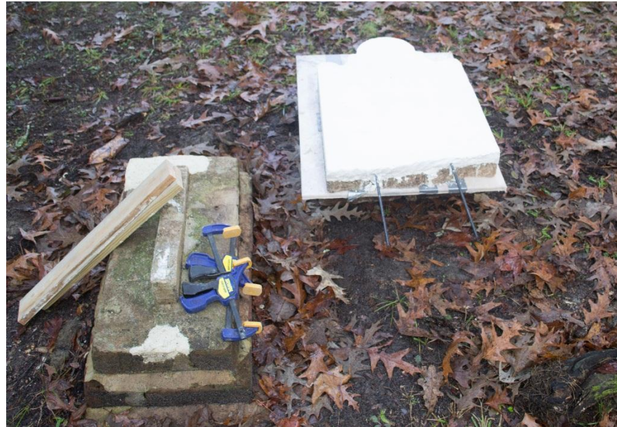
Rods are inserted into the base and epoxy applied between base and tablet
