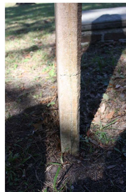
Cracks running down south elevation. Similar cracks also run down north elevation.
