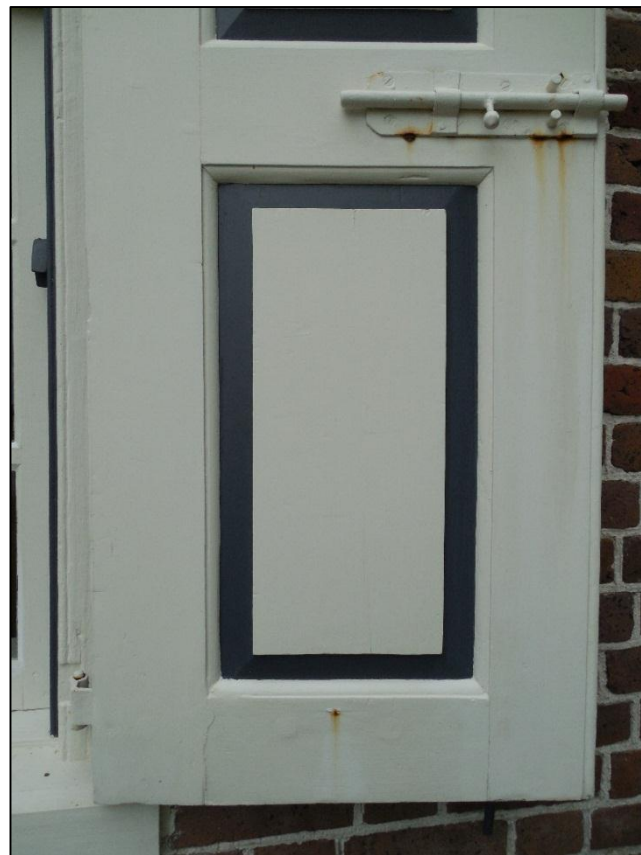
Detail of shutter showing paint scheme and bolt
