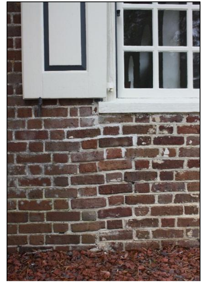
This is a current photograph of the Northeastern corner. This corner failed; most likely due to the arched window.
