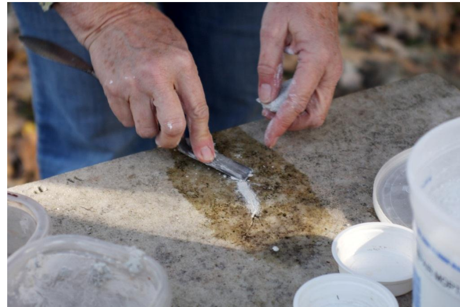
Applying Jahn to crack on ledge stone
