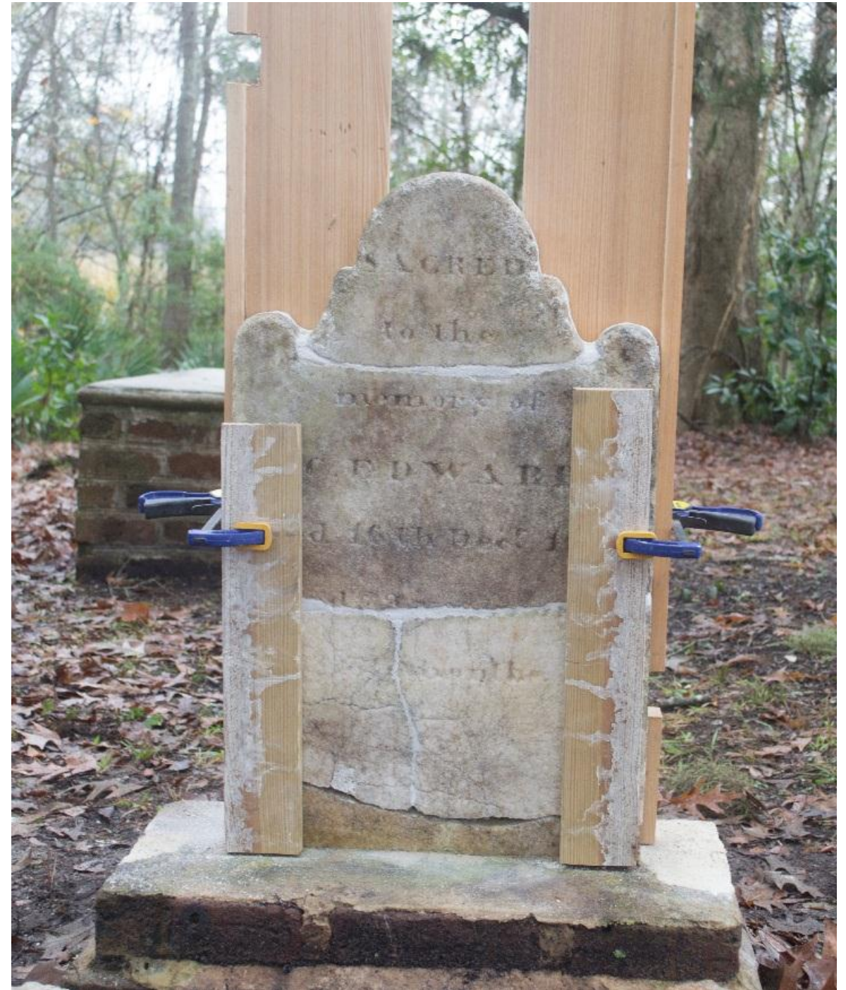
Finished result, boards soon removed once stable.
