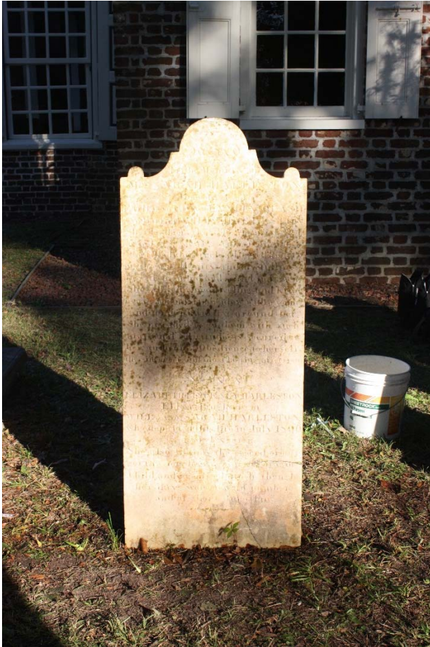
West elevation after cleaning. Staining and biogrowth are greatly reduced.
