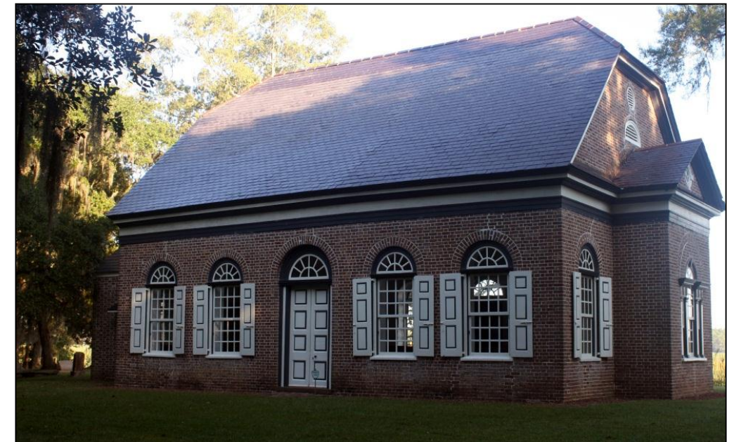
Jerkin head roof as seen from the south façade
