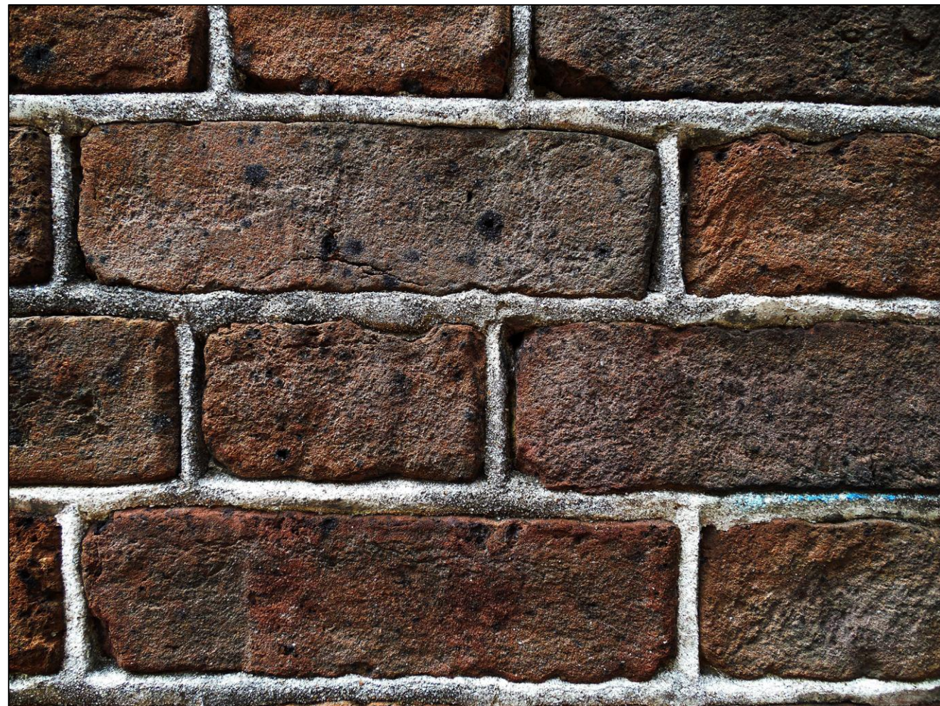
Above is a detail of the bricks. The masonry walls are constructed in a Flemish Bond Pattern with a ribbon joint.
