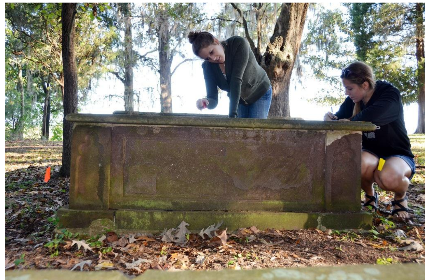
Applying Jahn to crack on ledge stone
