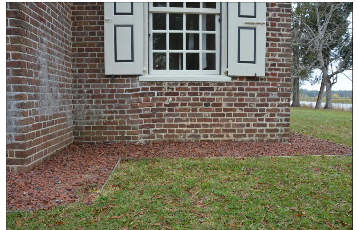
The NE corner as it is today. The French Drain surrounds the perimeter of the building.
