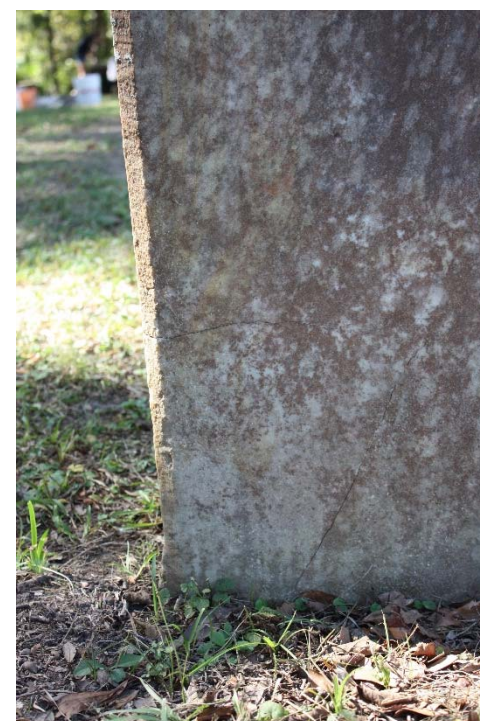
Monument is out of plumb, leans toward the east. (north elevation)
