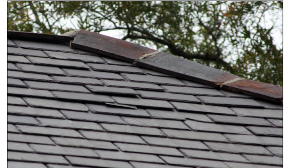
A detail of the ridge cap on the vestry.
