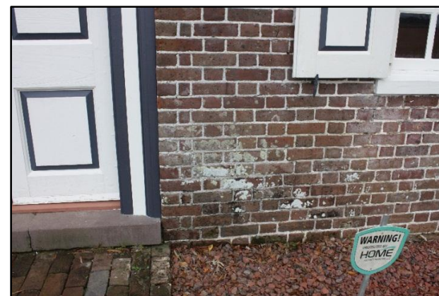
There is bio-growth present on the perimeter of the building.
