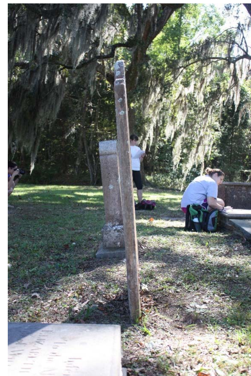
Monument is out of plumb, leans toward the east. (north elevation)
