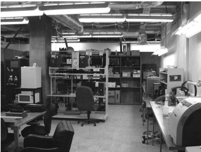
This existing space contains data servers, work spaces, and storage. Dedicated spaces would be given to each of these functions in their new locations on the renovated 2nd floor.
