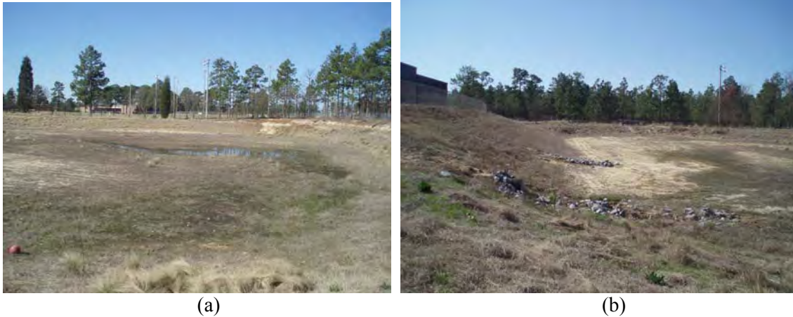
Figure H. 6. (a) Infiltration pond at North Springs Elementary school and (b) Drainage from the school's rooftop (background) and parking lot (foreground).
