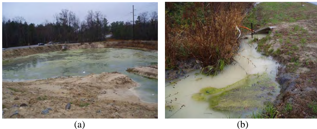
Figure 6.19. Site F-RRI-28 (a) soil needs to be stabilized and (b) sediment laden outflow from the stormwater pond.
