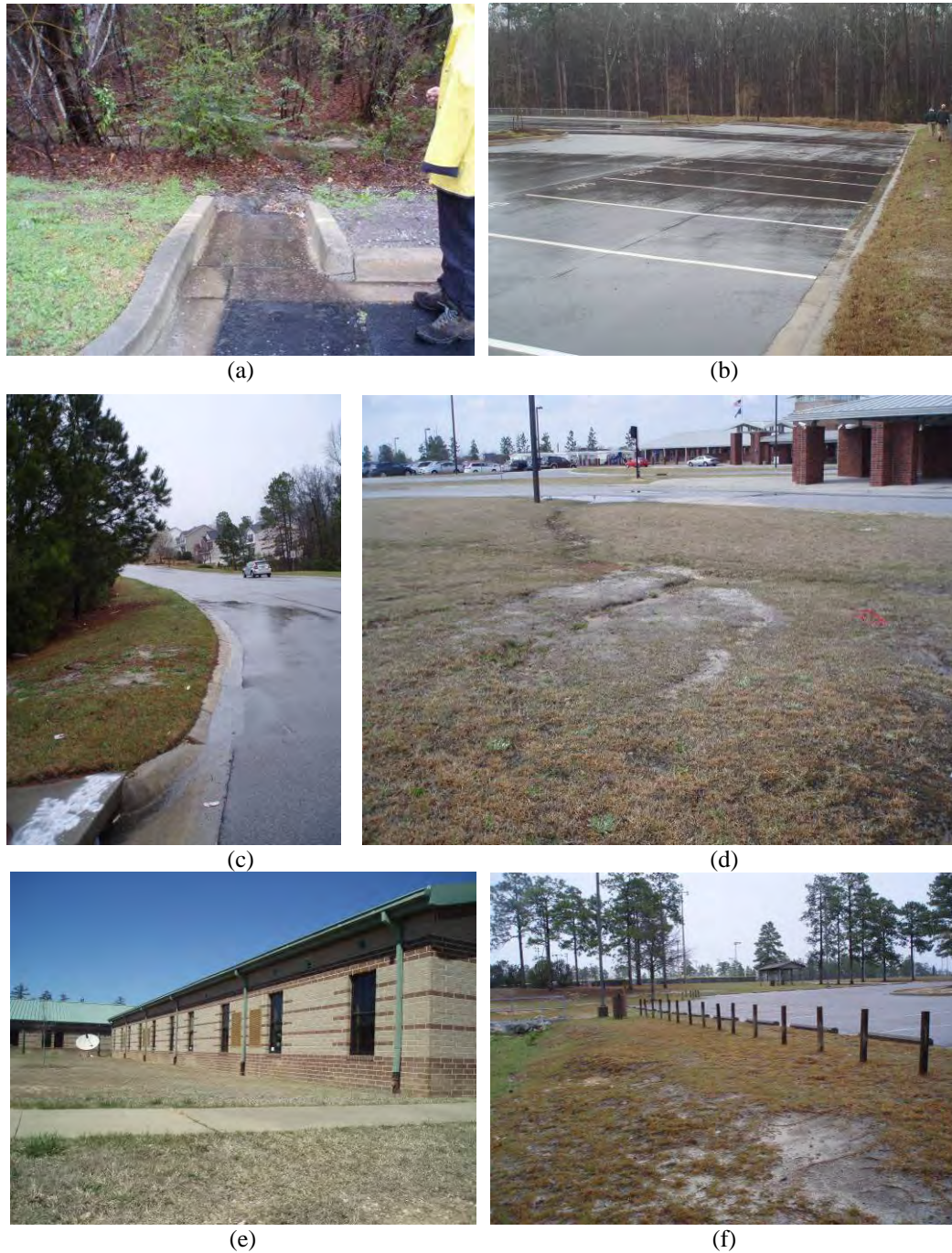
Figure 3.3. Stormwater retrofit opportunities. (a) Untreated business park parking lot runoff travelling directly to stream (H-RRI-24B); (b) untreated school parking lot runoff travelling into forested area (I-RRI-17); (c) opportunity for a roadway retrofit in a residential neighborhood (G-RRI-201); (d) proposed location for a bioretention area at a school (E-RRI-34); (e) downspout disconnection opportunity at a school (K-RRI-06); and (f) proposed location for a bioretention area to capture parking lot runoff from a park (G-RRI-38).
