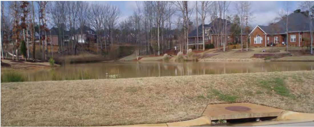
Figure H.1. Wet pond in need of maintenance. Also, a no-mow zone should be established around the pond perimeter.
