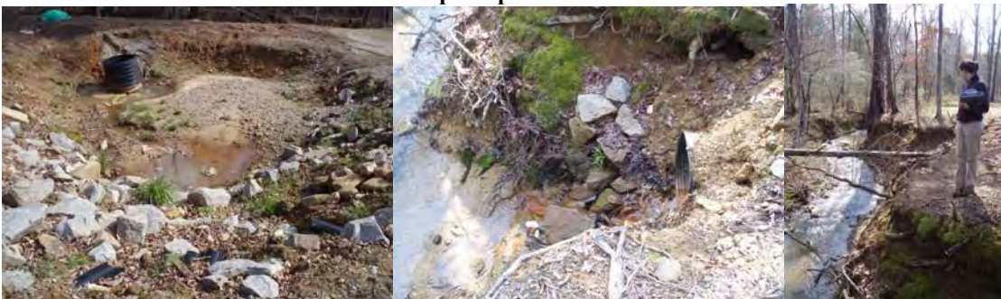
Figure H.2. Third pond in series which is undersized, badly eroded, and on the verge of failure. Stabilization and repair are needed to prevent blow-out of this pond into Beasley Creek.
