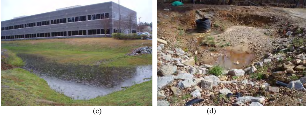
Figure 3.2. Poor functioning stormwater management practices. (a) erosion in a neighborhood dry pond (F-RRI-35); (b) stormwater pond with unstable drainage area (C-RRI-19B); (c) flood-control pond at business park with no water quality control (H-RRI-200); and (d) undersized neighborhood dry pond (A-RRI-21A).
