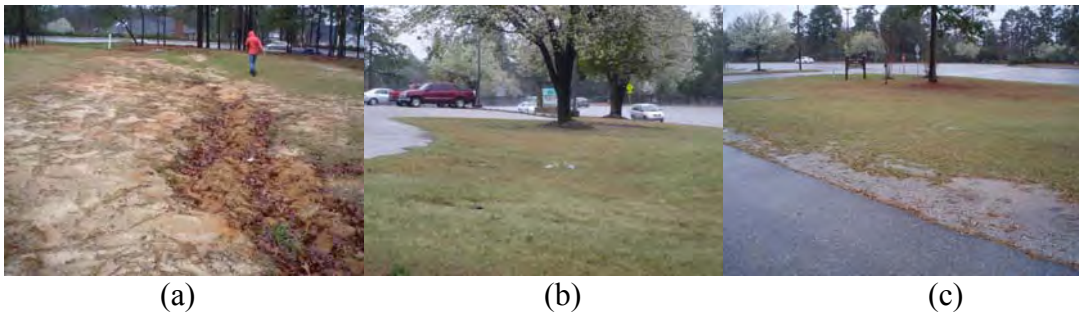
H.5. (a) North Spring Park eroded swale carries untreated stormwater runoff from a parking lot into the storm drain system and (b & c) Proposed locations of bioretention facilities.
