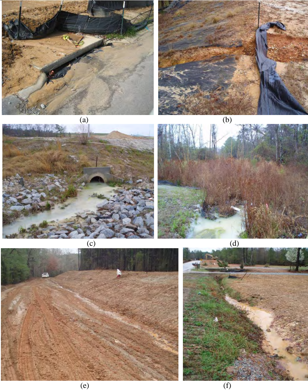
Figure 3.6. Erosion and sediment control problems found during field work. (a) Poor ESC at a subdivision construction site (E-ESC-2); (b) failing ESC at an inactive construction site (H-ESC-1); (c&d) sediment export from an abandoned sediment pond (F-ESC-2); and (e&d) poor ESC along utility line construction (B-ESC-2) and (B-ESC-1).
