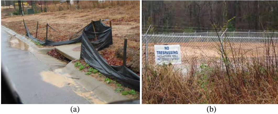
Figure 6.36. (a) Poor ESC practices at Hastings Point development (I-ESC-2) and (b) new development without ESC at Whitaker Container Service (I-ESC-1).
