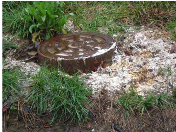
Figure 6.35. Evidence of sewage overflow in the Highland Forest neighborhood.
