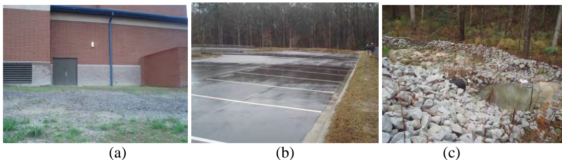
Figure 6.32. (a) Downspouts at site I-RRI-17; (b) southwest corner of lot drains most site; and (c) rip-rapped stilling basin discharging stormwater into nearby forested area.
