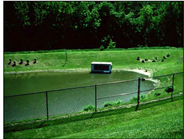
Figure 1: Wet Storm Water Pond
