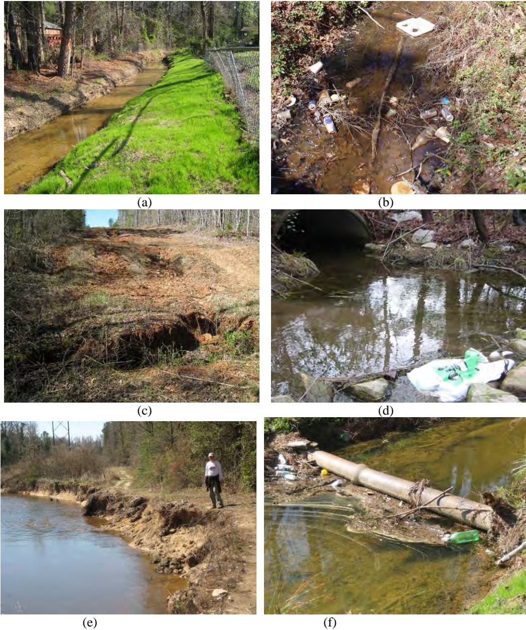
Figure 3.7 Stream restoration opportunities. (a) mowed and fertilized stream edge (L-RCH-5) located in neighborhood L-NSA-3; (b) trash including plastic bottles, wrappers and cups in G-RCH-10; (c) erosion impacts associated with utility crossing (J-ER-11); (d) fertilizer bag in stream in neighborhood G-NSA-2 (G-TR-2); (e) utility corridor located above stream reach K-RCH-13 contributing to bank erosion and impacted buffers; (f) sewer utility across stream acting as trash barrier (L-RCH-5).
