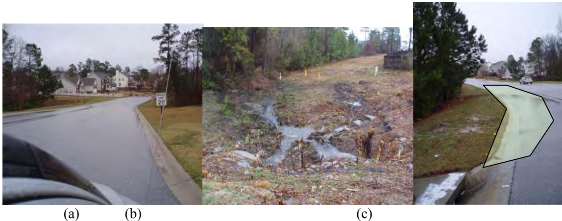
Figure H.12. (a) Alderston Rd. conveys untreated stormwater runoff to (b) a tributary of Upper Crane Creek. (c) Proposed retrofit location.
