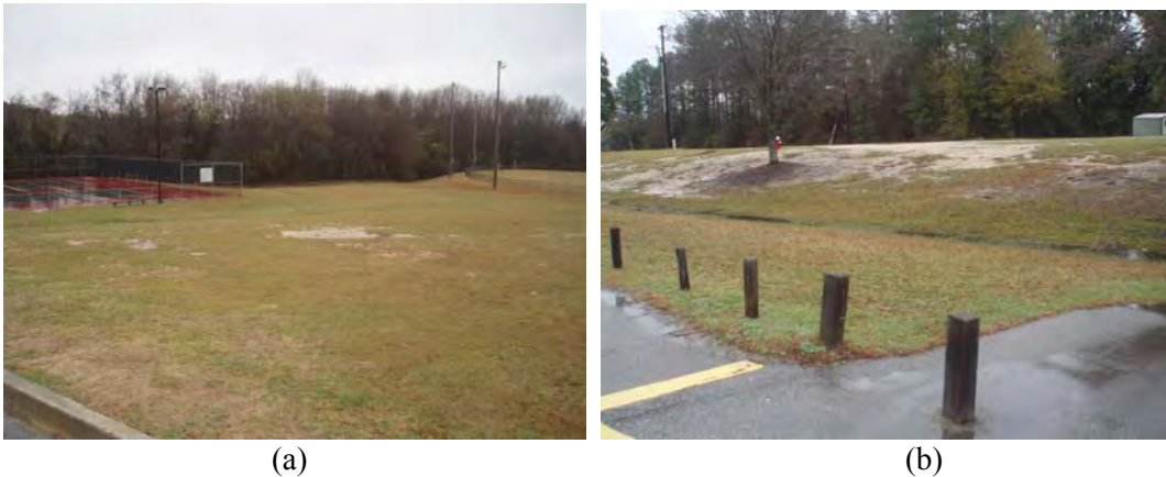
Figure H.10. (a) Much of the runoff at the Medowlakes Recreation Center drains via sheetflow to a nearby buffer and (b) An existing swale at the site could be enhanced with plantings.
