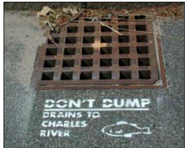
Figure 1: Storm Drain Marking
