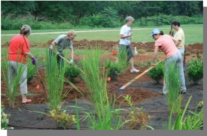
Mulching a rain garden.
