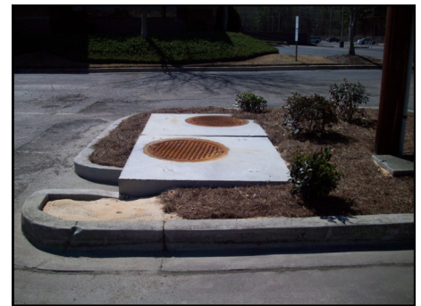
Right: Catch basins installed as part of capital improvement projects at Windsor Lake Blvd. (top) and Farrow Road (bottom).
