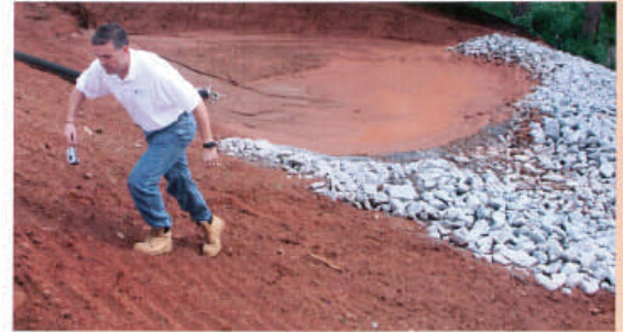
Cal Sawyer inspects a construction site for compliance with erosion prevention practices to water quality in the state's streams and lakes.
