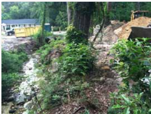
Sediment flowing into a stream from a construction site near Lake Katherine.
