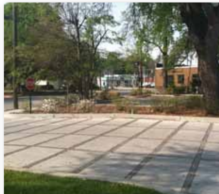
Pervious pavement at Sumter Pediatrics lets the parking lot drain to the soil beneath.
