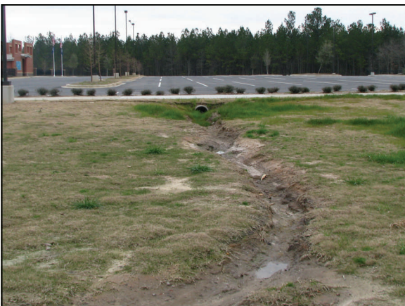
Erosion from parking lot run-off at Patriot Park
