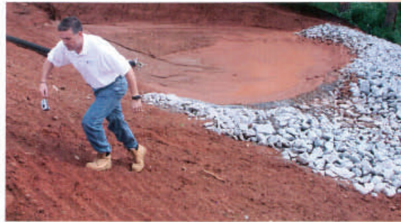
Cal Sawyer inspects a construction site for compliance with erosion prevention practices to water quality in the state's streams and lakes.
