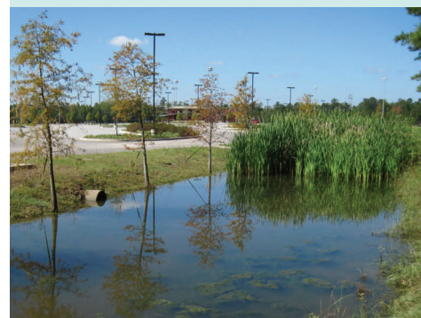
Constructed wetland at Patriot Park
