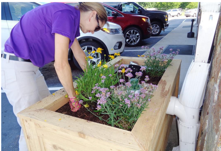
▲ Extension Agent Terasa Lott helps install a downspout planter box at Raceway Ford of Darlington.
