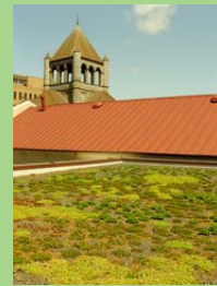
Green roof, Circular Congregational Church
