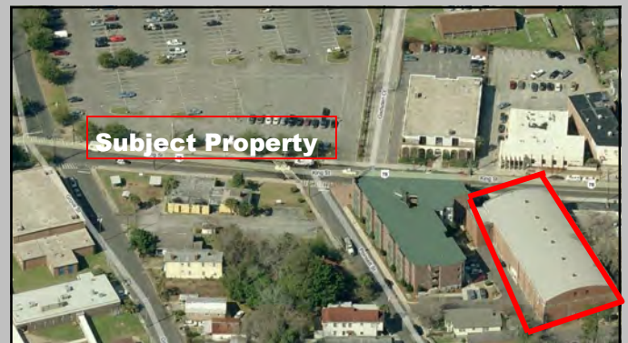
Subject Property Looking West
