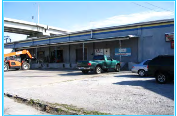
Dock high loading with four 8x8 overhead doors
