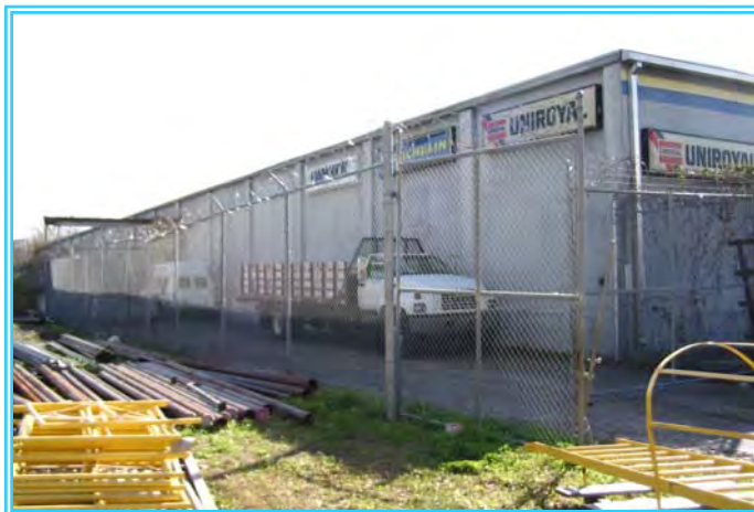
Fenced side yard with loading dock & overhead door
