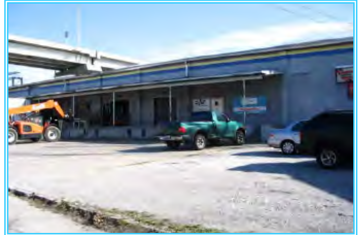
Dock high loading with four 8x8 overhead doors
