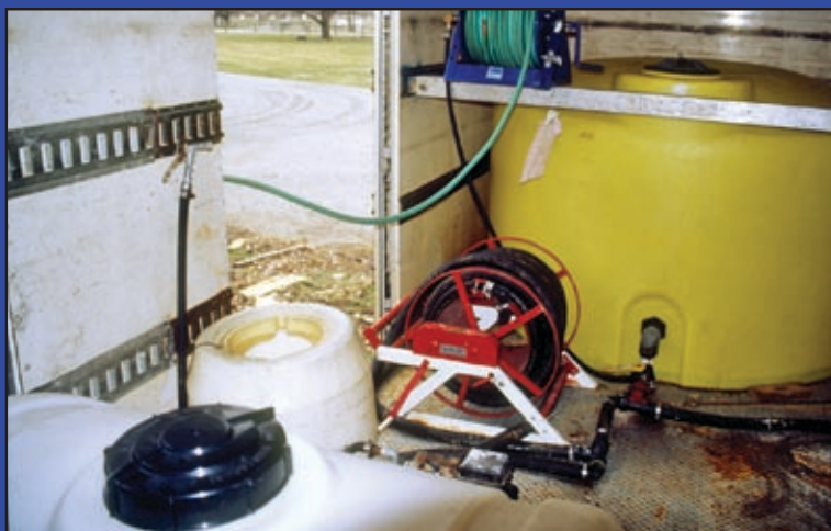
The yellow poly tank inside this trailer is secured by a metal bar.
