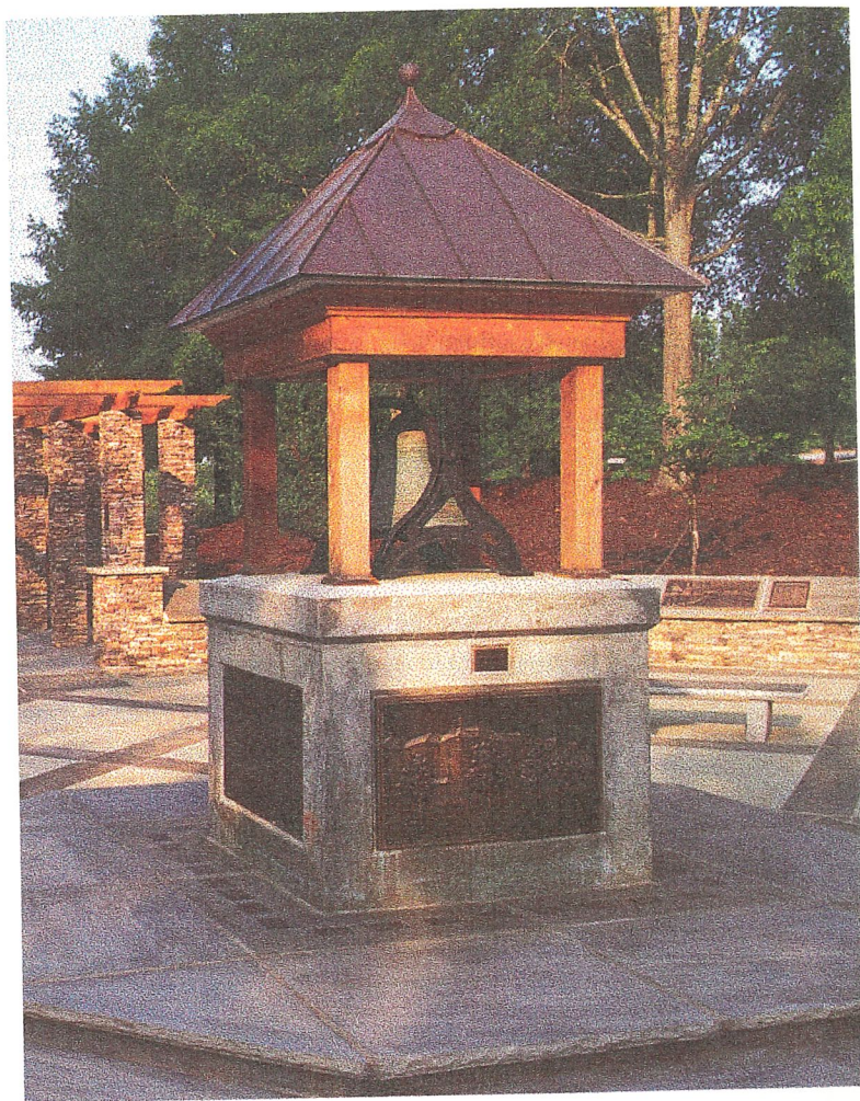
The Guardroom Bell Structure
