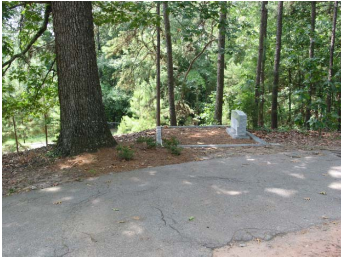
Recent coping installation under 36" Red Oak
