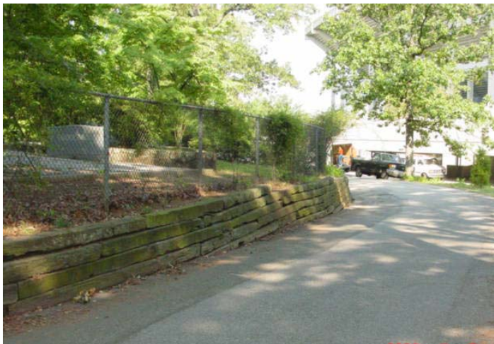
Existing cross-tie retaining wall
