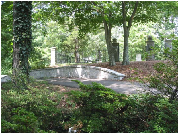
New retaining wall installed in 2000
