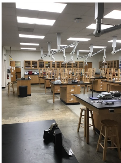
Snorkels on articulated arms used in a general chemistry lab.
