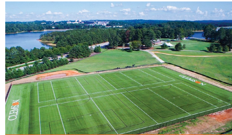
THE NEWLY INSTALLED LOCONTE FAMILY FIELD
